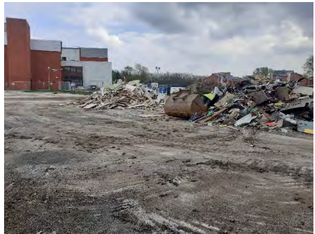
19.04.23 – Stockpiles of removed wastes from college building pending sorting and recycling.
