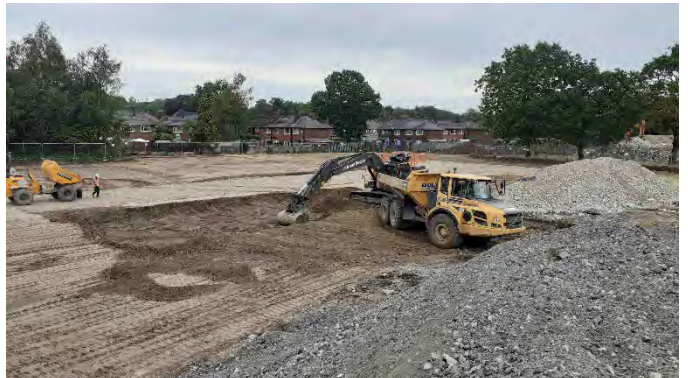
18.07.23 – Cut and fill works taking place in the centre
