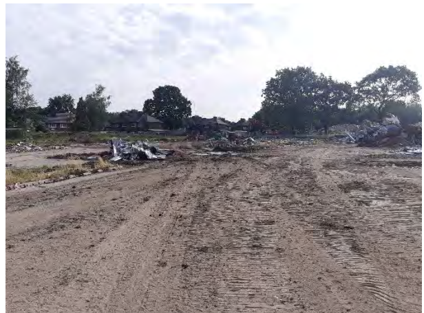
22.06.23 – Northern view prior to breaking out of hardstanding.
