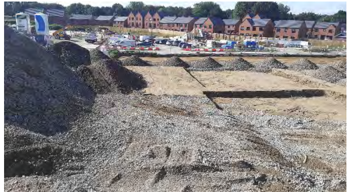
01.09.23 – Southern view from aggregate stockpile in the east of the site.
