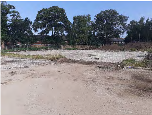
22.06.23 – Northwest corner following bungalow demolition.
