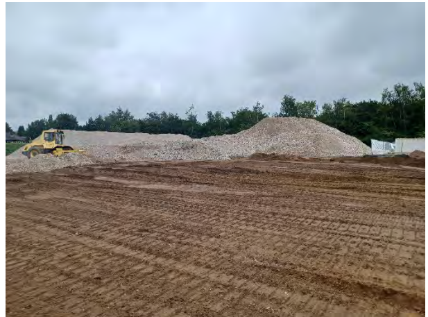
24.08.23 – rolling of replaced soils in the centre/east
