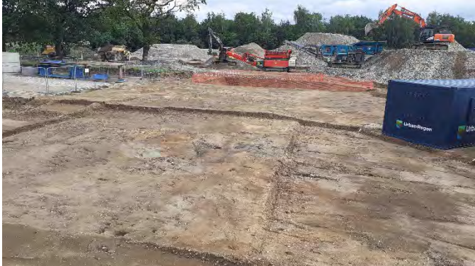
15.08.23 – Completed area in the centre / west.
