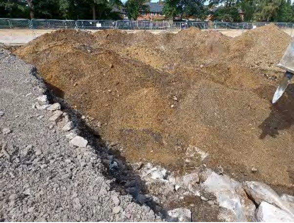
26.07.23 – Inspection of soils during turnover in the centre / west adjacent to completed area
