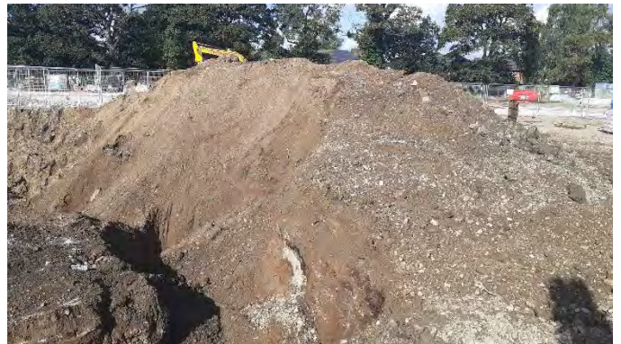
01.09.23 – Temporarily side cast soils to exposure relict foundations. Soils observed by SGP and consisted of natural sands.
