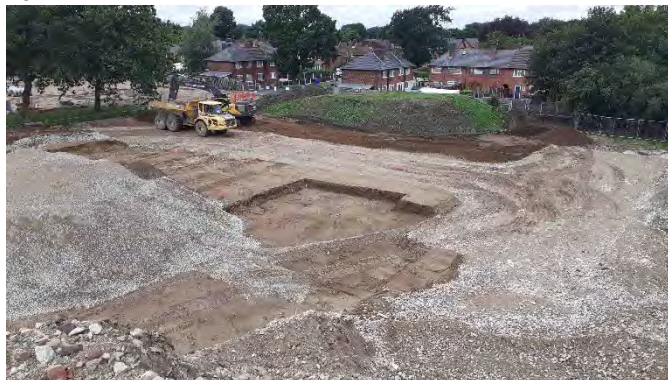
15.08.23 – Northern view from the eastern end of the site.
