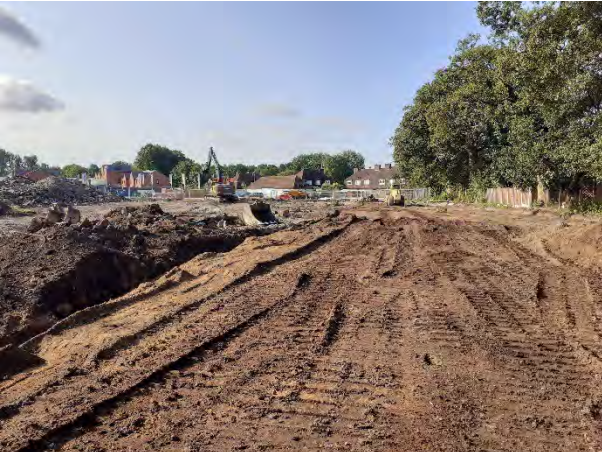
29.06.23 – Area of completed turnover in the north.
