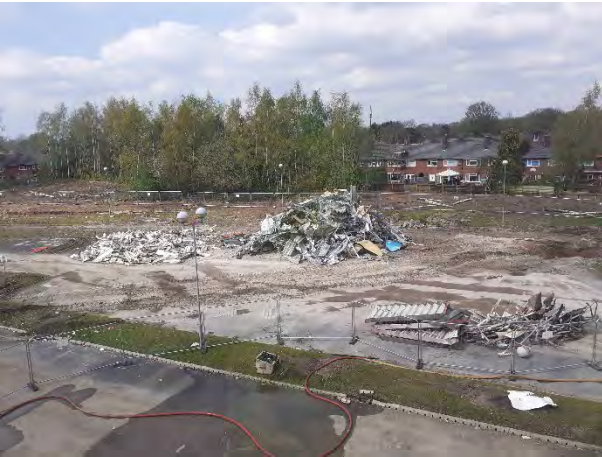
19.04.23 – Northern with stockpiles of recyclable wastes recovered from college building.
