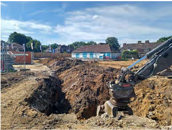
06.07.23 – Turnover of made ground in the southwest
