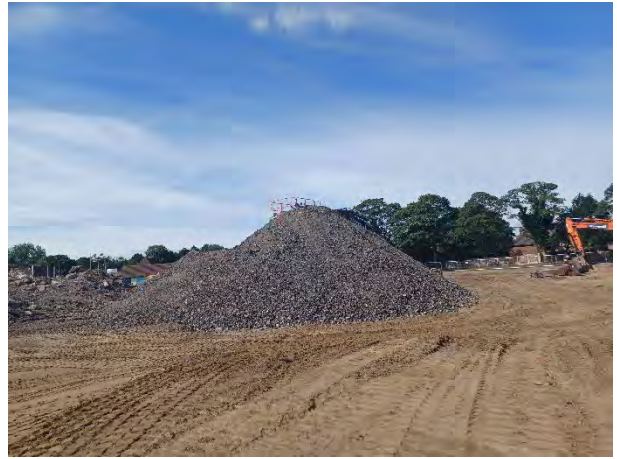
06.07.23 – Stockpile of generated aggregate (MOT) in centre of the site (crushed behind).
