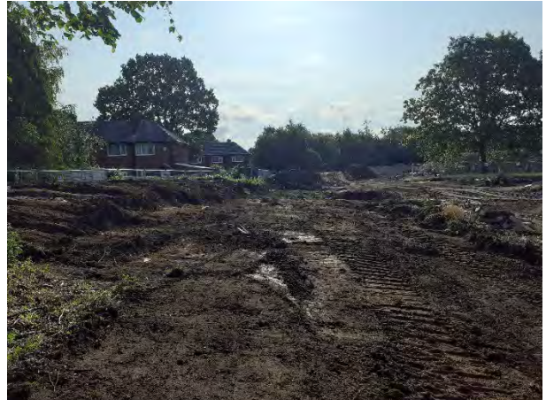
29.06.23 – Topsoil stripped and recovered from embankment / landscaping area in the north.
