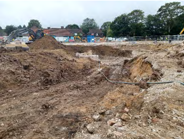
24.08.23 – Ground conditions observed during removal of relict foundations.
