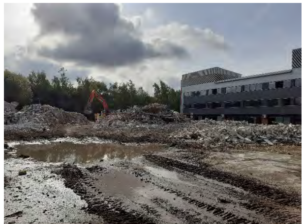
17.05.23 – Stockpiles of demolition material pending recover of metal (rebar)
