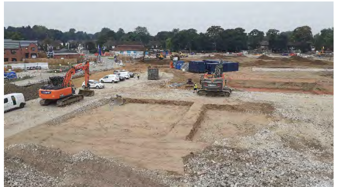
08.09.23 – Placement of aggregate in road box in the east.
