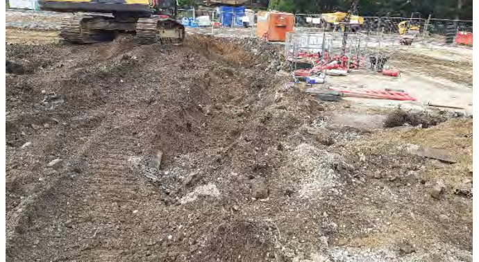
15.08.23 – Turnover of soils and removal of relict services in the centre/west.
