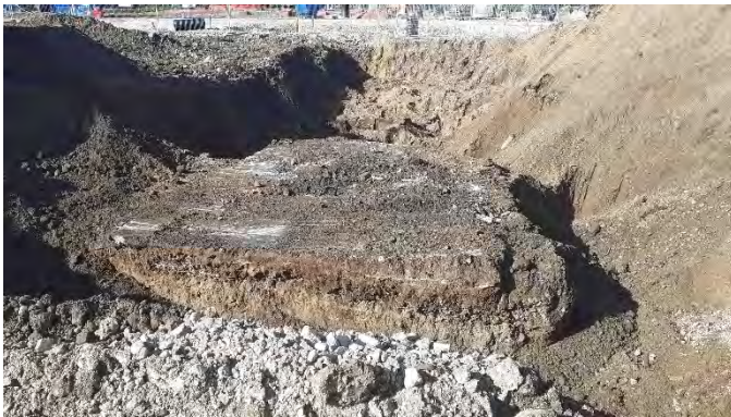
01.09.23 – Exposure of relict foundations prior to removal.
