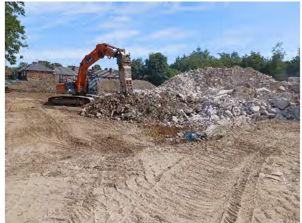
26.07.23 – Pulverising broken out hardstanding to recover metal rebar
