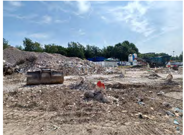
26.07.23 – southern area within footprint of former college building awaiting removal of foundations and turnover of soils.
