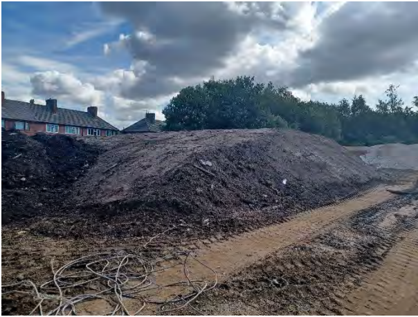
06.07.23 – Stockpile of site-won topsoil in the north.
