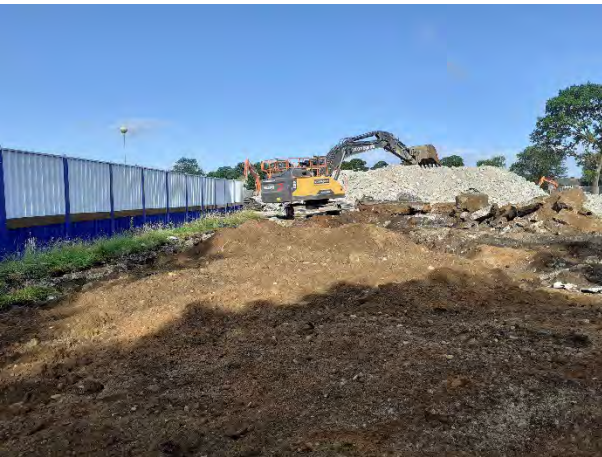
29.06.23 – Removal of relict foundations from former college and turnover of soils in the southeast
