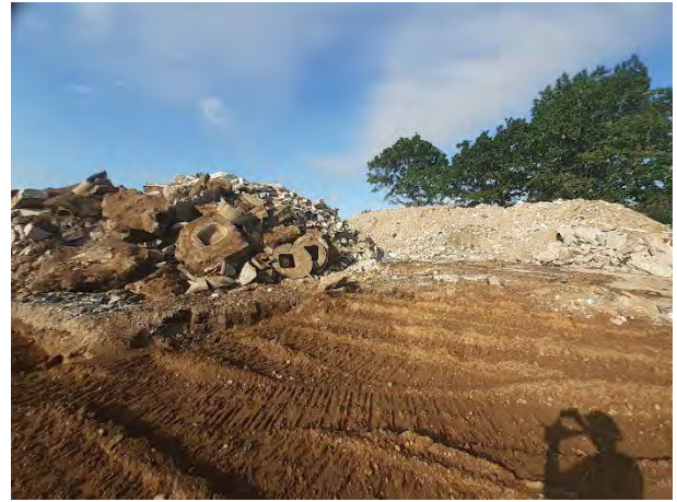
29.06.23 – Stockpiles of recovered hardstanding awaiting processing in the centre.
