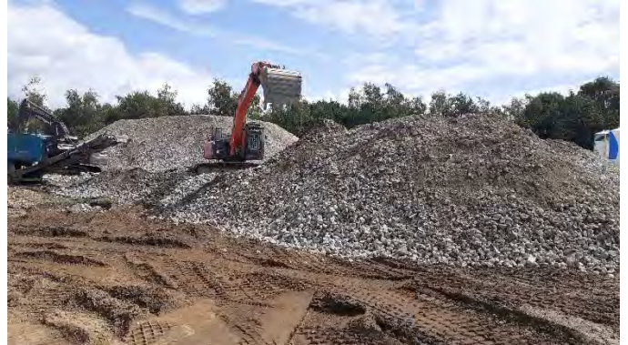
03.08.23 – 6F2 Aggregate stockpile (~4,500m 3 )
