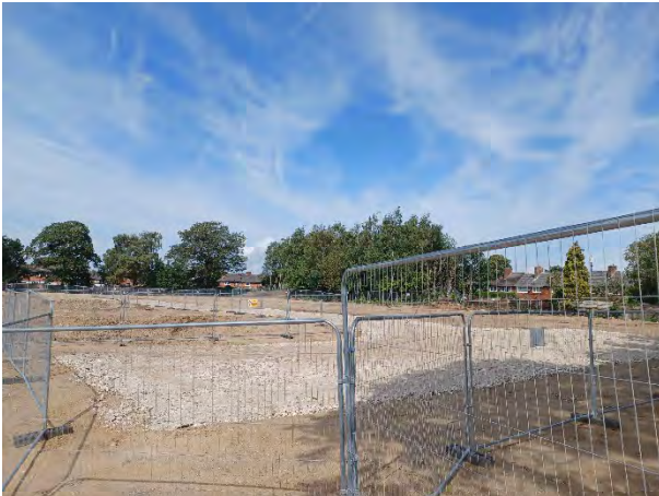
26.07.23 – Preparatory works completed in the west and fenced off
