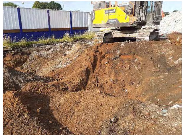
29.06.23 – Inspection of soils during turnover.
