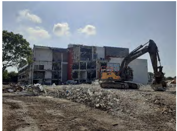
26.05.23 – Demolition of college building on-going.
