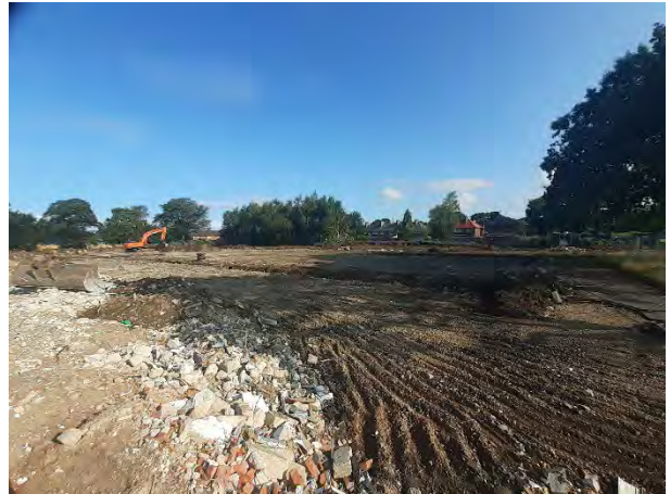
29.06.23 – Western view across the site following removal of surface hardstanding.
