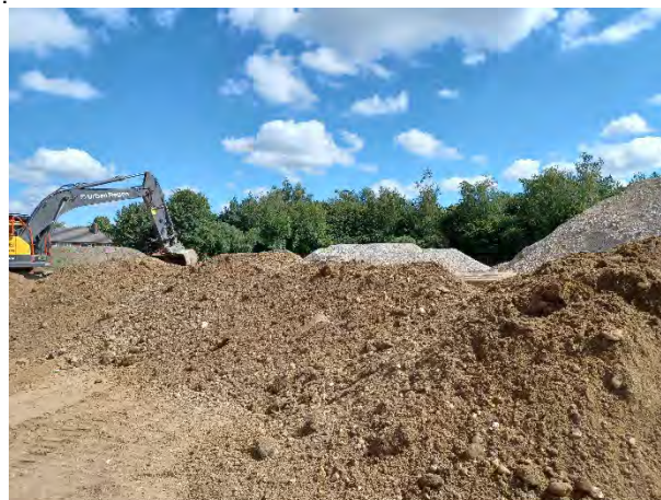
10.08.23 – Cut and fill works in the centre.
