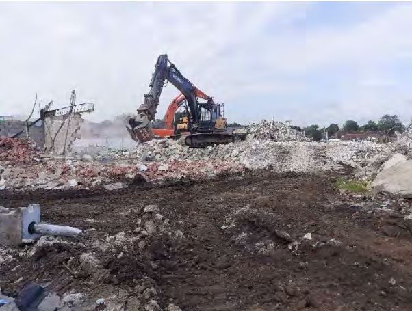
22.06.23 – Final demolition works of remaining college building walls.
