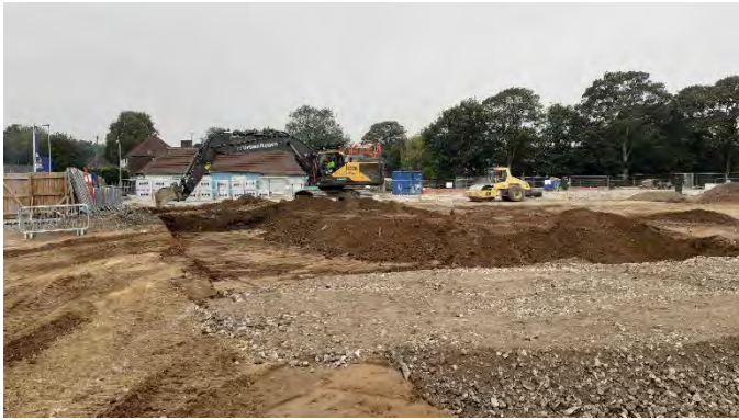
08.09.23 – Cut and fill works taking place in the centre.
