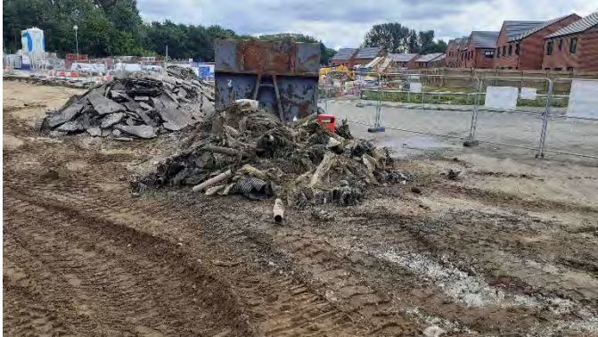
15.08.23 – Waste materials recovered during recent turnover works awaiting off-site disposal.
