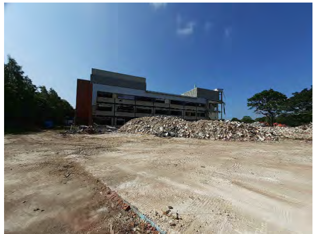
26.05.23 – College building with northern wing demolished.
