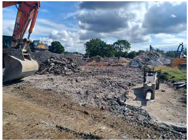
06.07.23 – Areas of exposed made ground following removal of surface slab.
