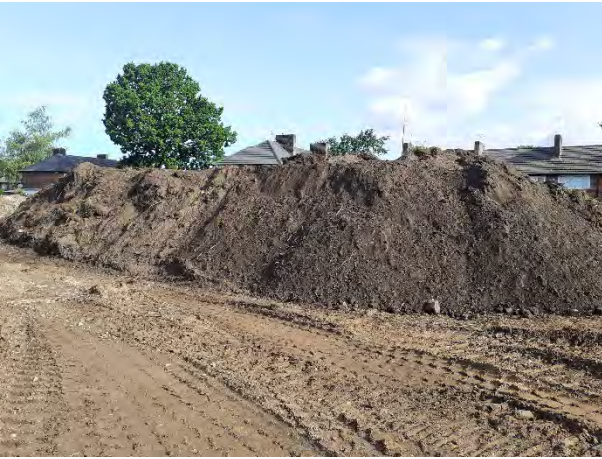
29.06.23 – Stockpile of recovered topsoil awaiting testing.
