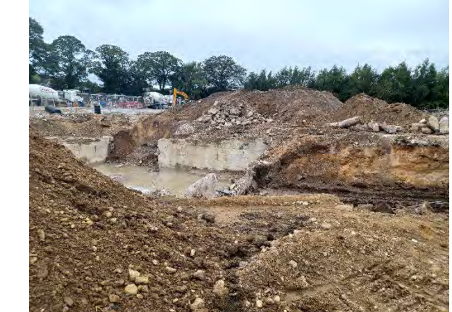
24.08.23 – Exposing of relict foundations (original college building) under former car park area in the west.
