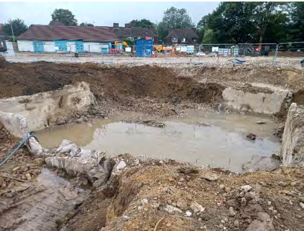
24.08.23 – Former foundations prior to removal
