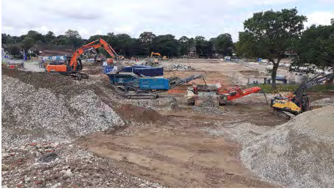
15.08.23 – Processing hardstanding in the centre.
