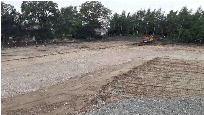
18.07.23 – Placement of site-generated aggregate in the northwest complete.
