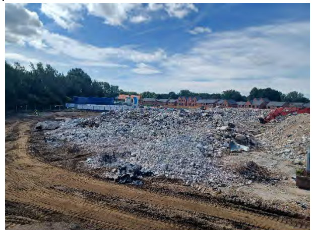
06.07.23 – Stockpiles of recovered hardstanding in footprint of former college building pending processing.
