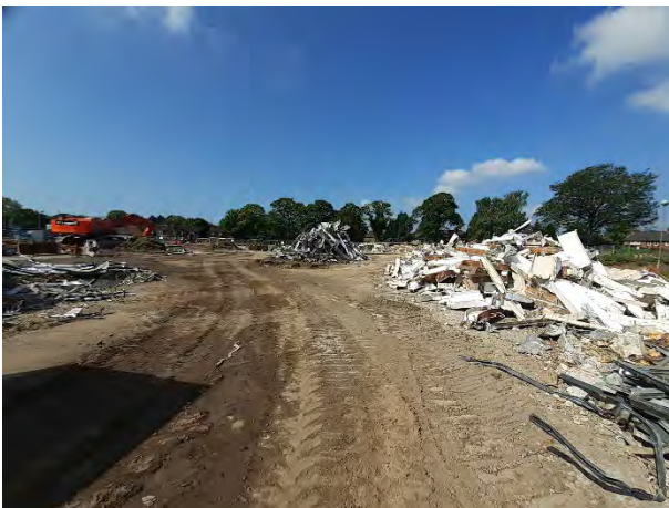
26.05.23 – Hardstanding removed from external areas of building and stockpiled pending processing. Stockpiles of recovered wastes pending recycling.
