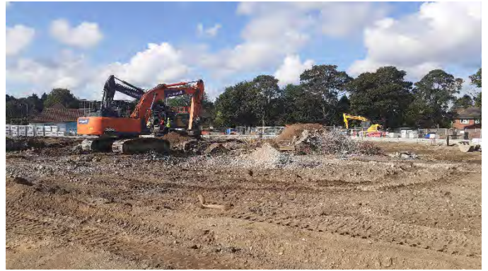
01.09.23 – Removal of relict foundations / turnover of soils.
