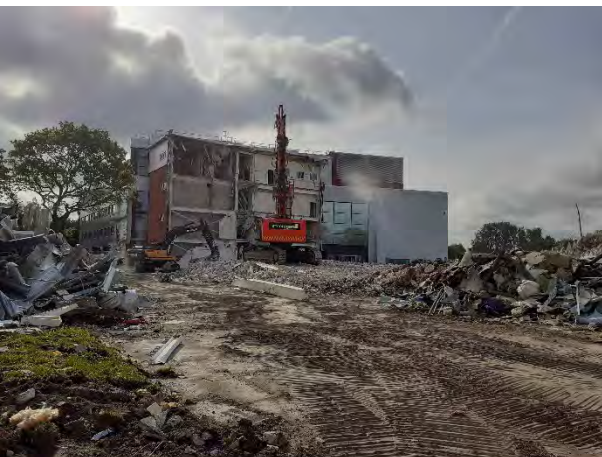
17.05.23 – Demolition of college building
