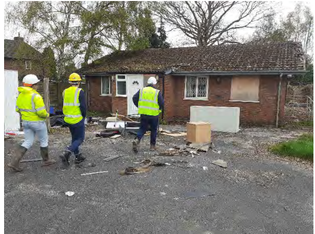
19.04.23 – Inspection of former bungalow in the northwest of the site.
