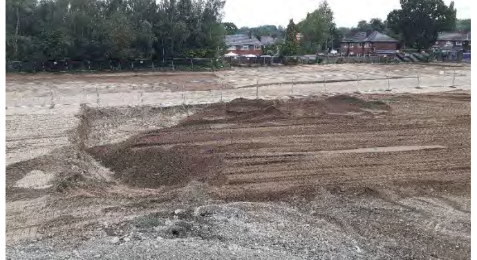
18.07.23 – Placement of site-derived fills in the east as part of cut and fill works.
