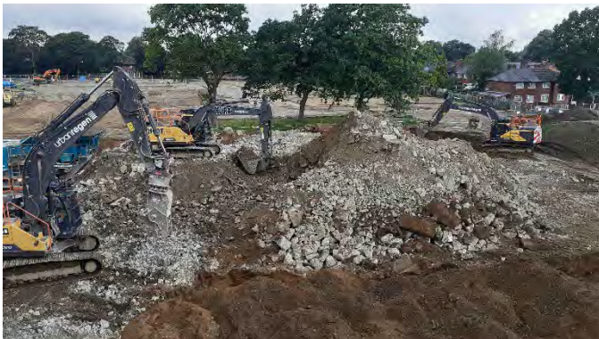
03.08.23 – Breaking out of relict foundations of former college building
