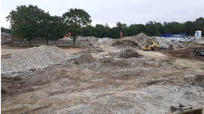
18.07.23 – Stockpiles of aggregate (processed) and recovered hardstanding (unprocessed) in the centre.
