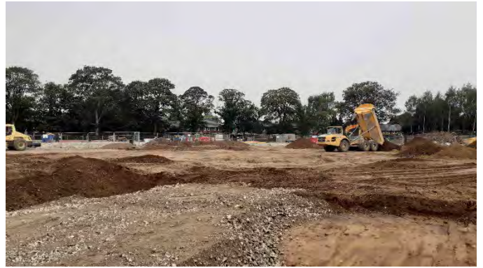
08.09.23 – Relocation of fill generated as part of cut works.
