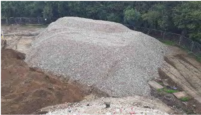
03.08.23 – Recovered aggregate stockpile (~1,088m 3 )
