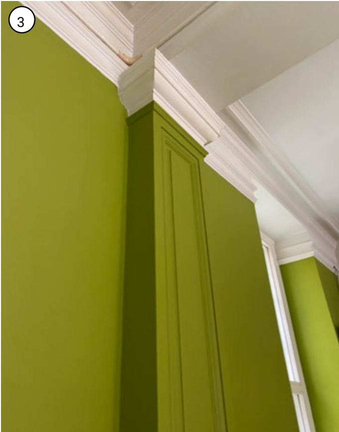
Original Plasterwork, to be retained or encased & protected for future reveal.
