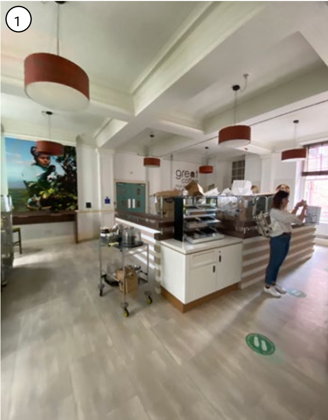
Original Downstand Beams - to be left exposed.
