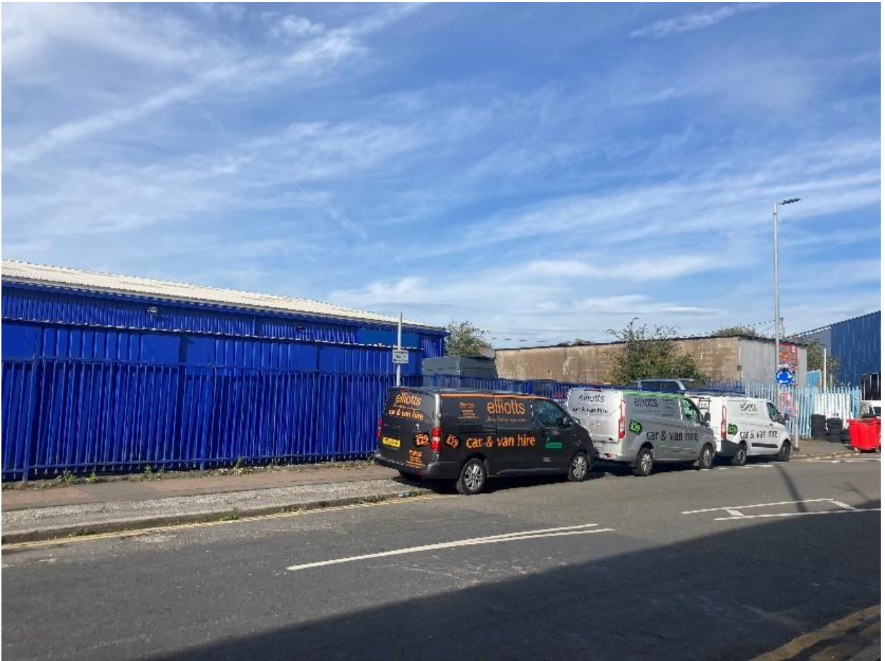
Figure 3.9 – View of the location of the proposed extension
