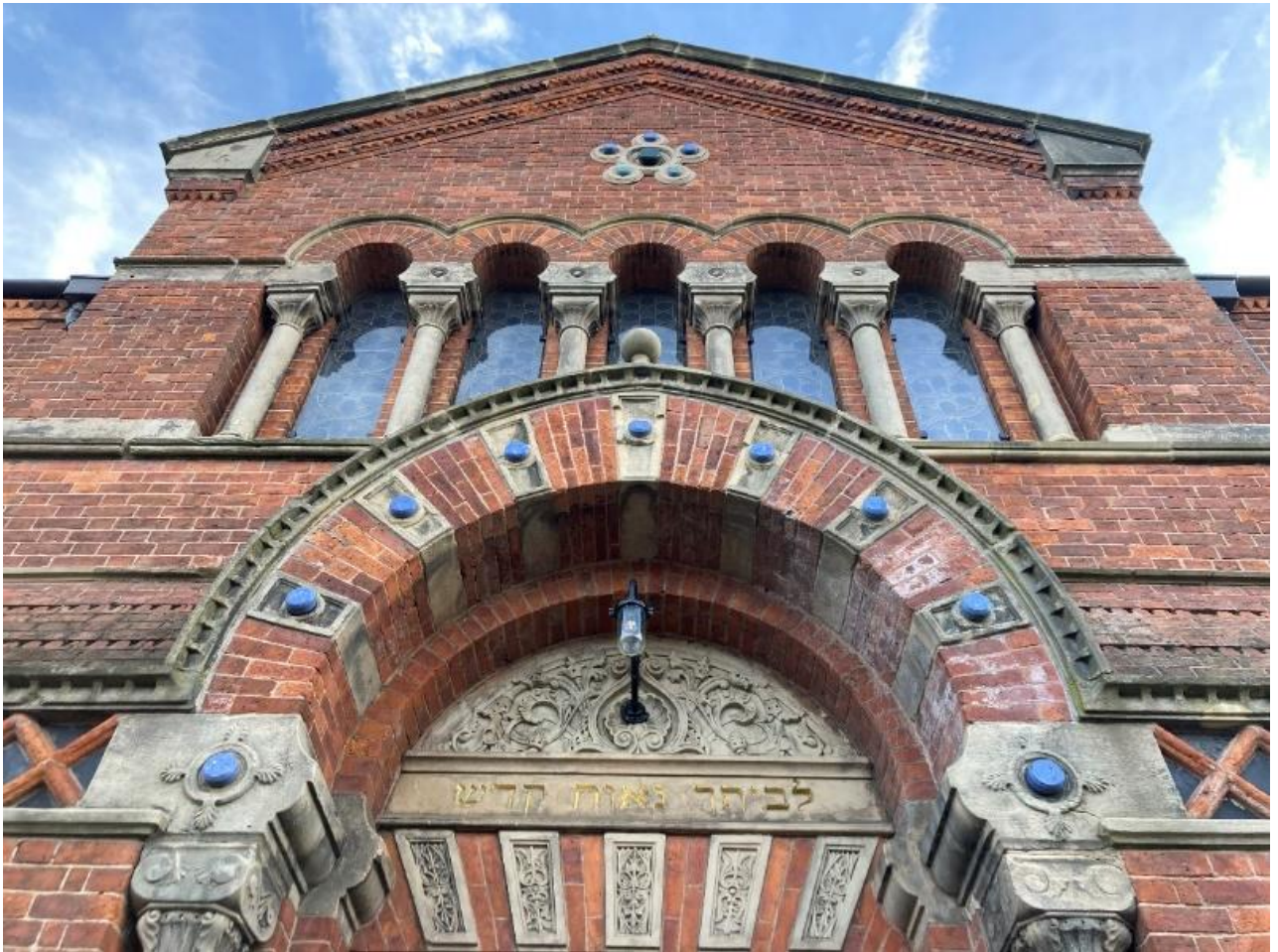
Figure 3.5 – detailing on the principal elevation of the synagogue
