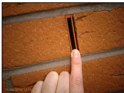
Figure 2: Weep hole with insert
