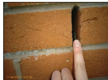
Figure 3: Weep hole without insert
