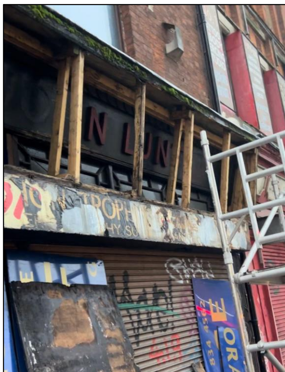
Figure 4: View of shopfront beneath existing fascia.
