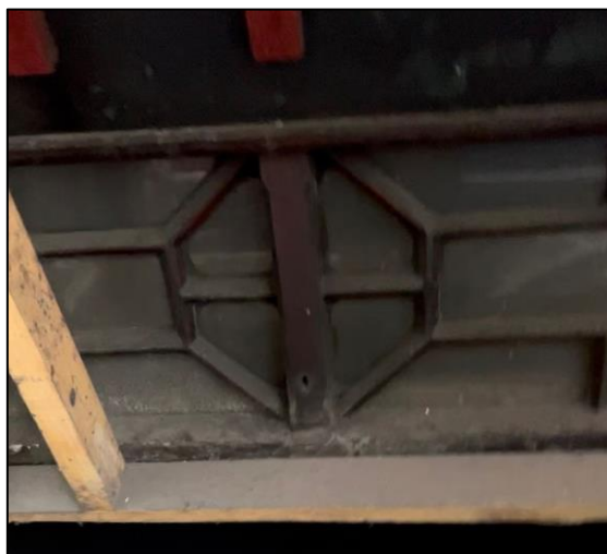
Figure 6: View of shopfront beneath existing fascia.
