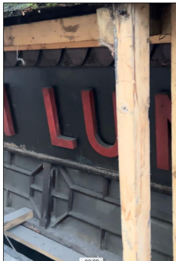
Figure 7: View of shopfront beneath existing fascia.
