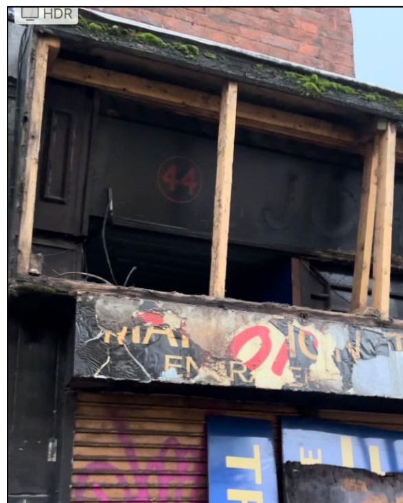
Figure 5: View of shopfront beneath existing fascia.
