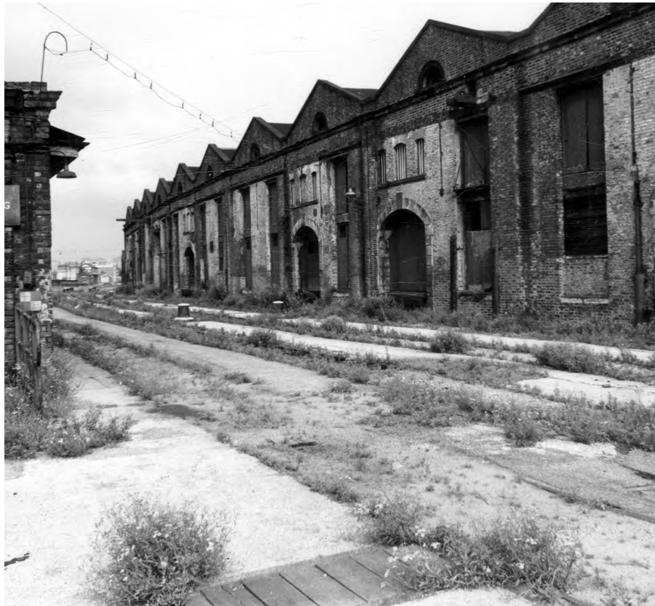
Figure 15 1830 Warehouse, 1979 © Manchester Libraries (m62976).
