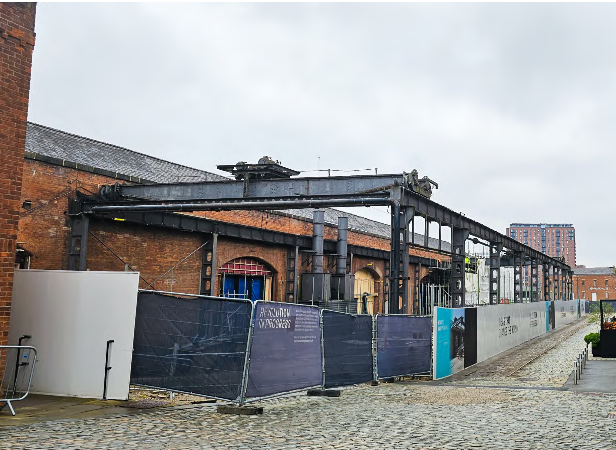
Figure 5 Power Hall North Elevation showing the Gantry Crane
