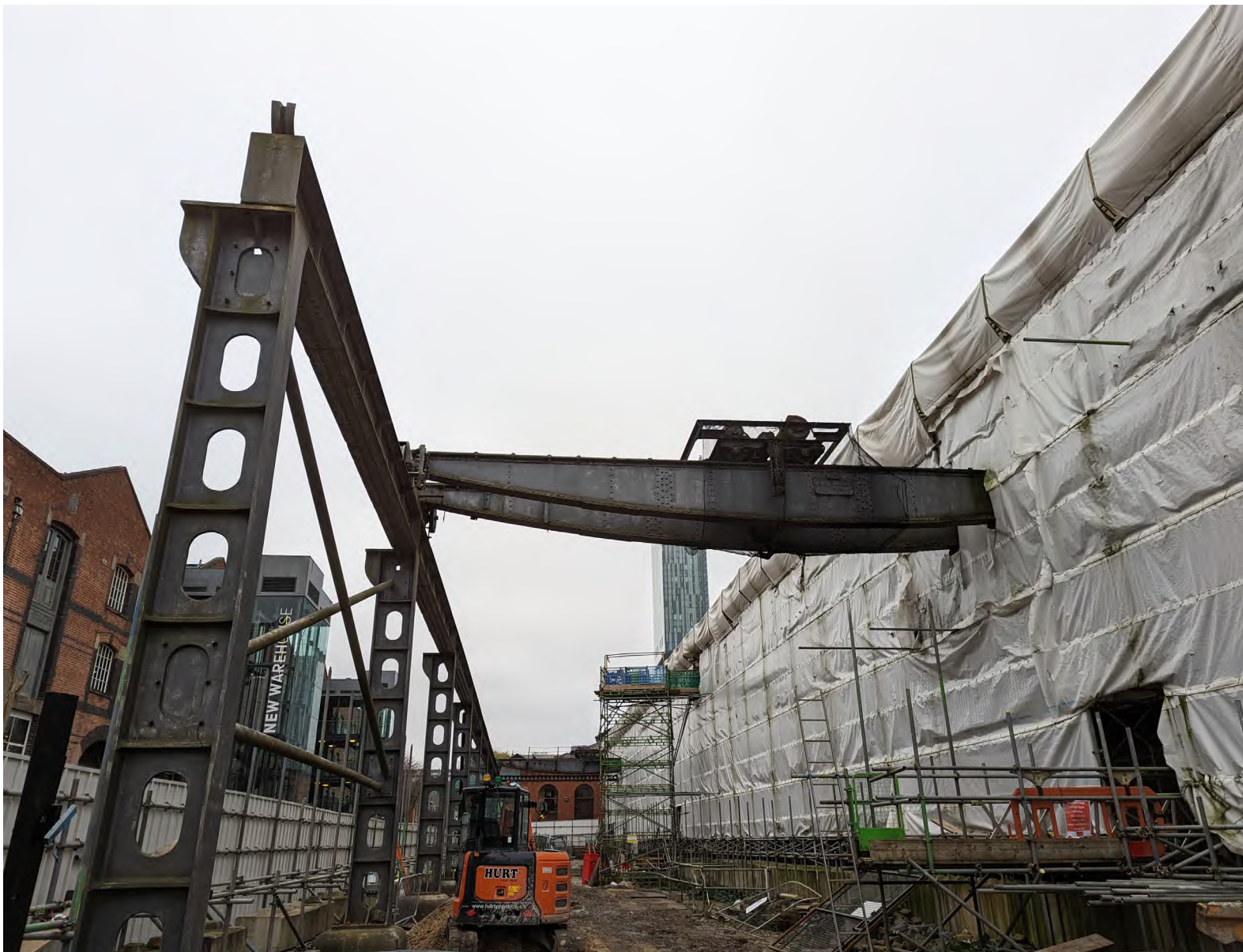
Figure 7 Gantry (view from west)
