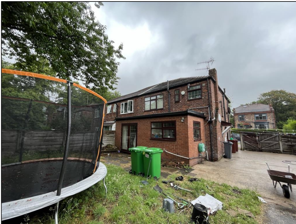
Figure 2. Rear of property
