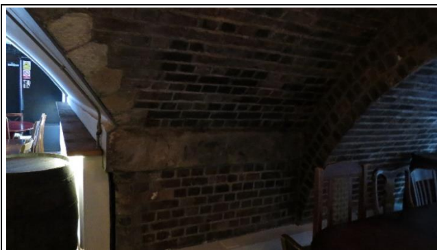
Detail of Arch Brickwork and Impost
