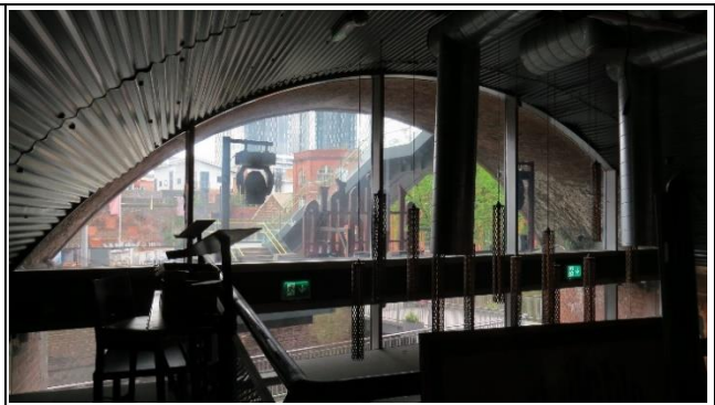
Ceiling of Arch 12 and Mezzanine
