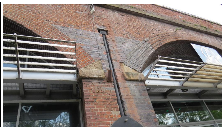
Detail of Arch Brickwork and Rainwater Goods
