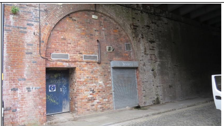
Grey Roller Shutter Entrance to Arch 1 Basement
