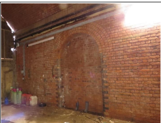
Bricked up Arched Opening to Arch 2
