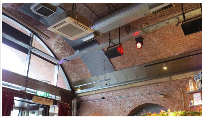
Remedial Works to West Side of Arch 7
