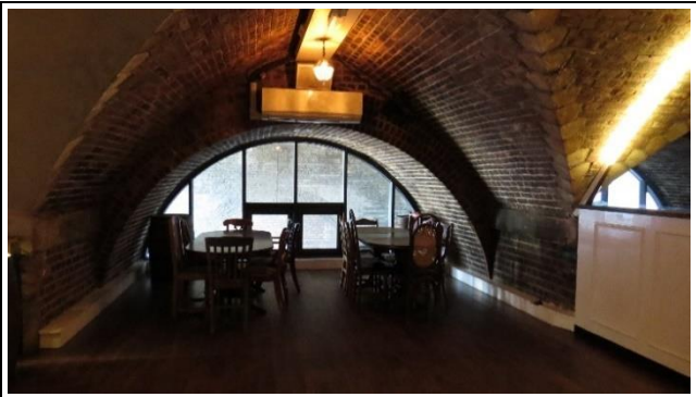
Arch 1- Area Over Century St Entrance
