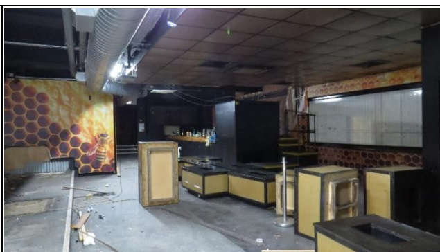
Basement Looking South
