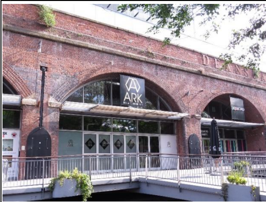
Front Elevation of Arches 5 & 6
