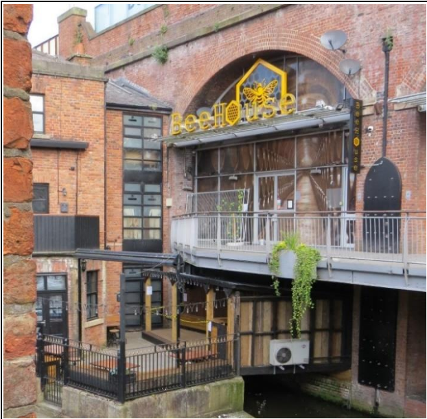
Front Elevation of Arch 2
