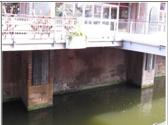
Absence of Basement
