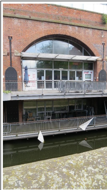
External Arch with Glazing
