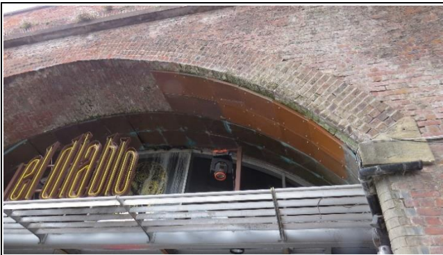
Copper Panels under Arch 11's Entrance
