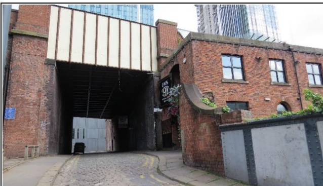
Viaduct with Bridge over Century Street
