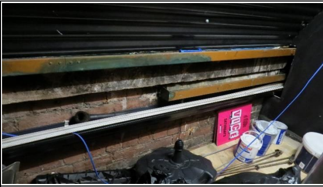
Supplementary Guttering and Ceiling Lining
