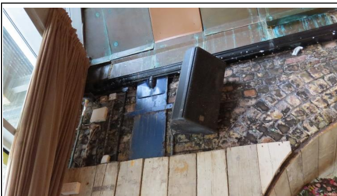
Concealing Boards Between Arches 7 and 8
