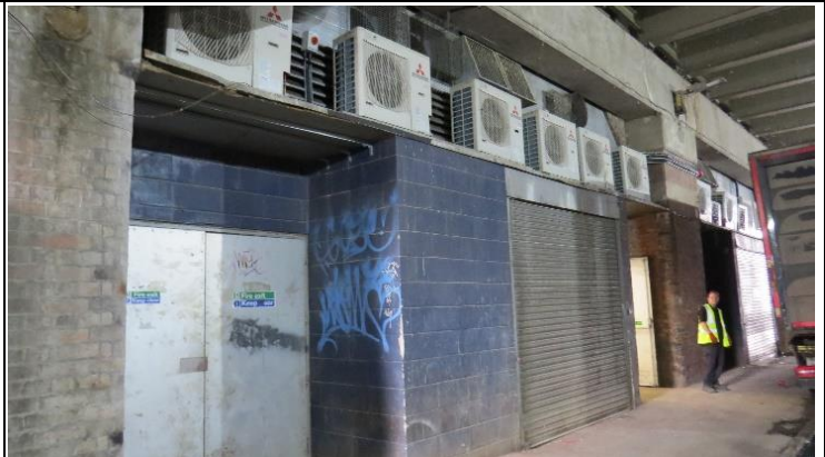
Rear Elevation of Arches 5 and 6
