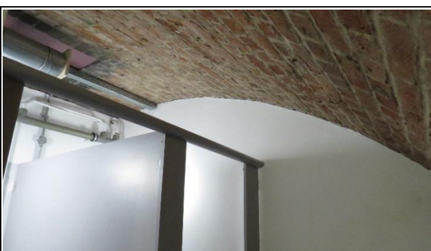
Vaulted Brick Ceiling of Southeast Arch
