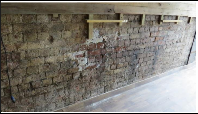
Timber Batons and Wall Lining
