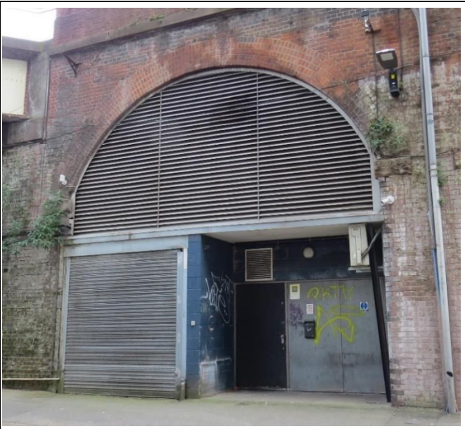
Rear Elevation of Arch 2
