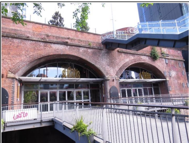
Front Elevation of Arches 11 & 12
