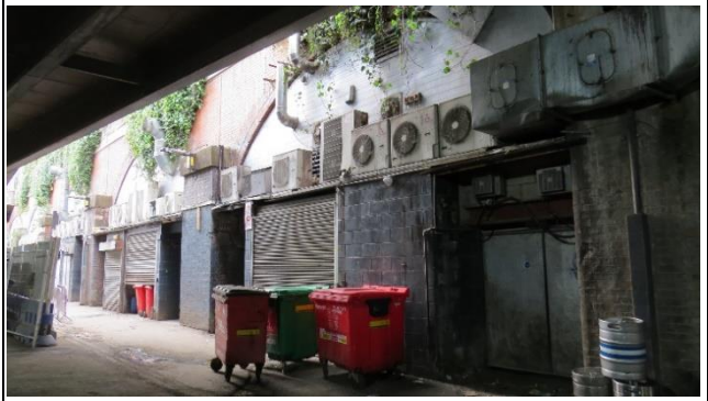
Rear Elevation of Arches 7 and 8
