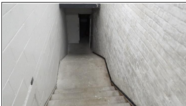
Arch 1 Stairs to Basement
