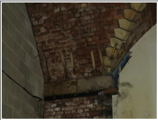
Detail of Blocking up of Crossvault Arches
