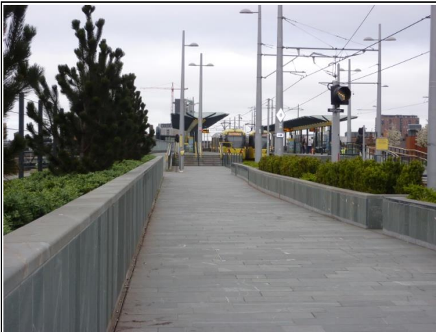
Pedestrian Walkway to Whitworth St. West
