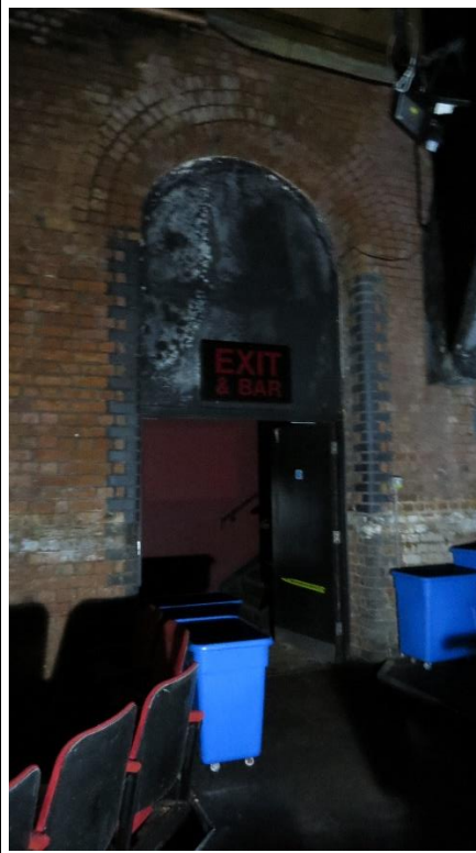
Internal Connecting Arch
