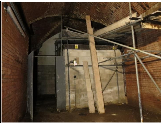
Breezeblock Staircase Structure under Crossvault
