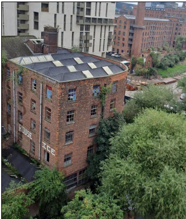
Figure 1: The roof of the south of the building from the multistorey carpark to the west.
