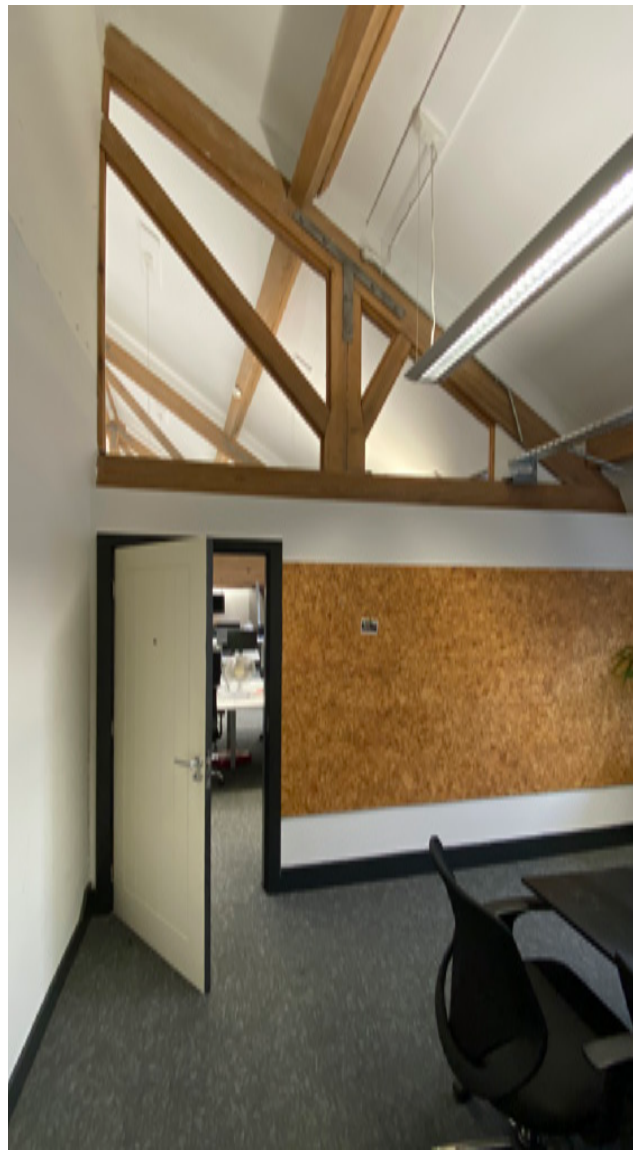
3.3.8 Partial height partition to the southwest corner. The wall to the left is partially part of the historic hoist core, with the section adjoining the door a later addition
