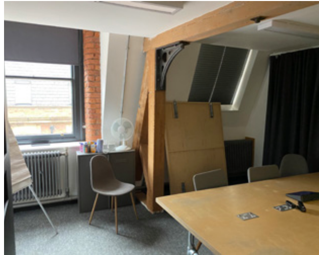
3.3.11 Indicative example of interior of meeting pods to the north outer wall. Historic elements include the timber supports, brackets, and brickwork around window reveals
