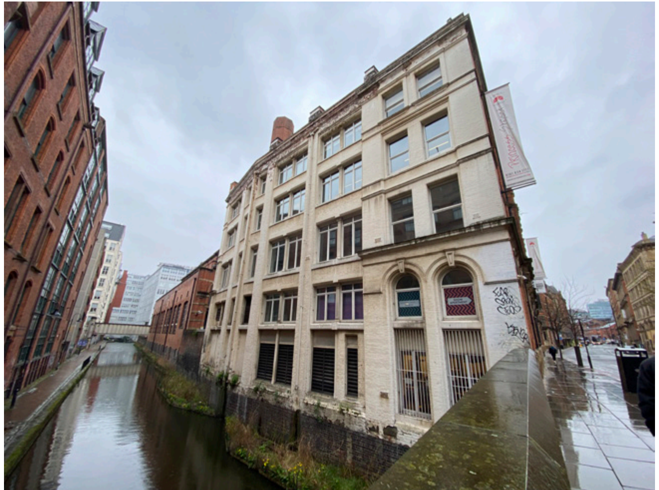
3.2.3 South return elevation of No.56 along the Rochdale Canal
