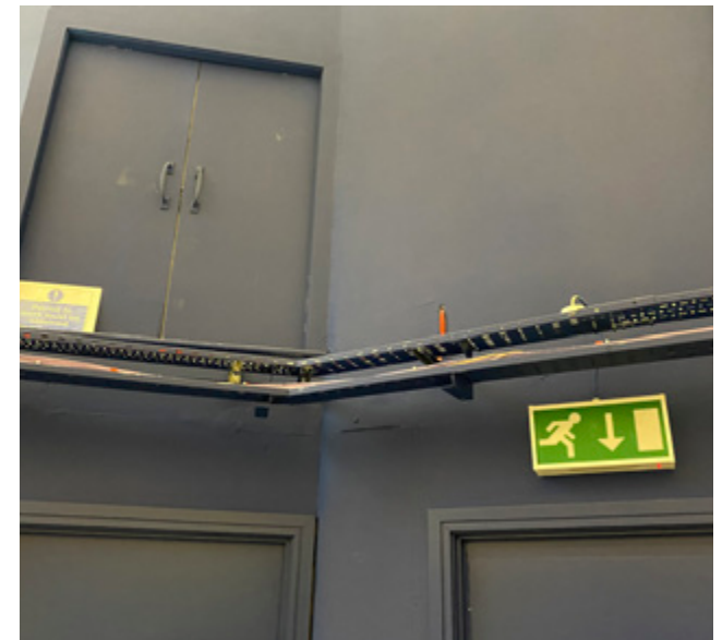
3.3.15 closeup of the south interior wall partitions, showing later canted addition to the earlier staircore wall
