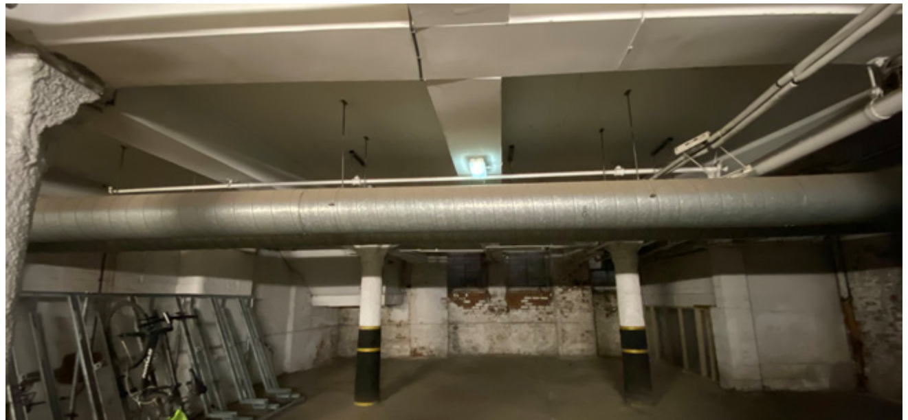
3.3.4 Basement showing columns and overboarded beams. Location for the proposed condensing unit to the far wall
