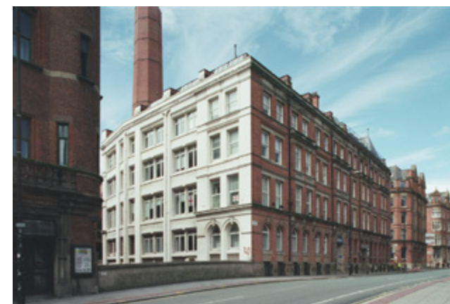
2.17 54 (R) and 56 (L) Princess Street, 2004 (Historic England)
