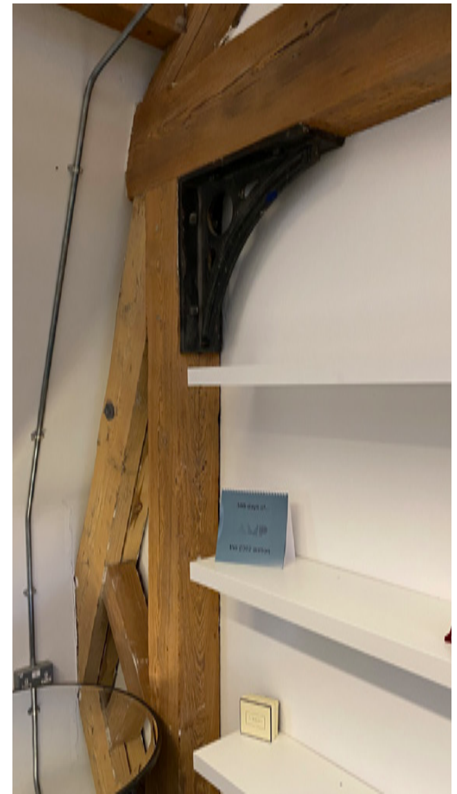
3.3.9 Indicative example of the timber supports with brackets, to the exterior of the southwest meeting room
