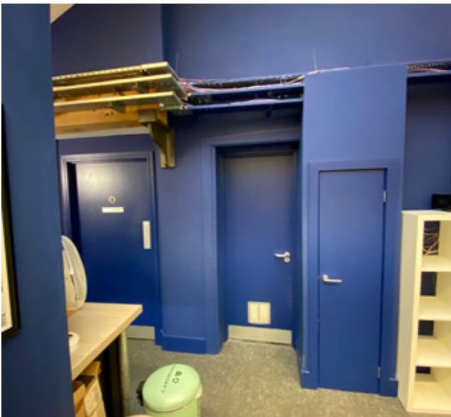
3.3.13 closeup of the south wall with partitions for toilets and the riser (central doorway)
