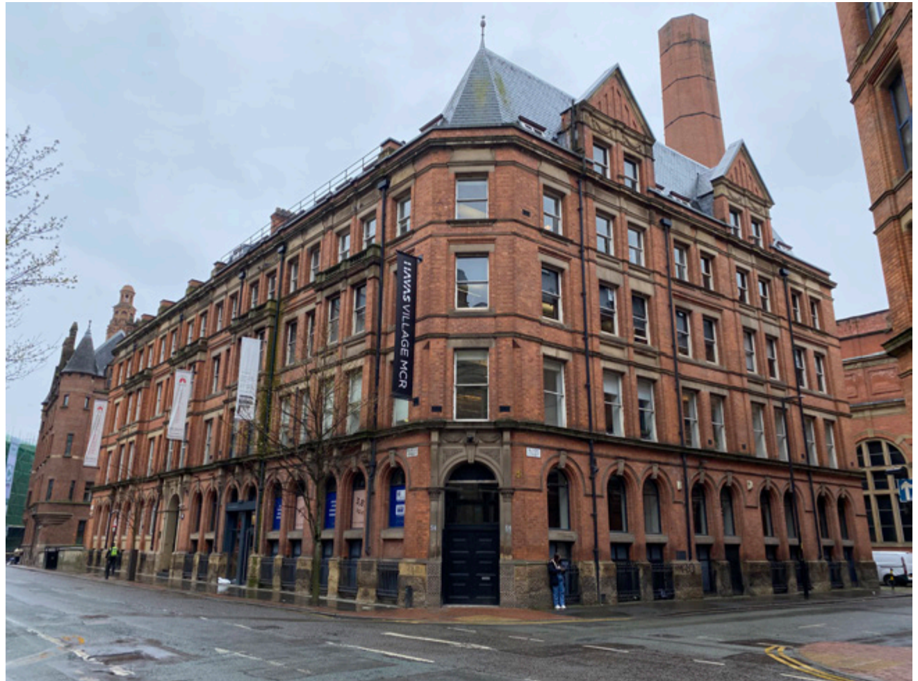
3.2.1 Front and north return elevation, with canted corner, at the junction of Princess and Bloom Streets, with chimney of the former electricity generating station behind
