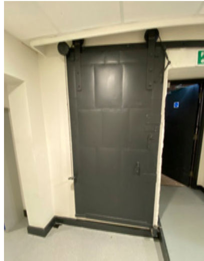
3.3.1 Historic door between the staircore and basement
