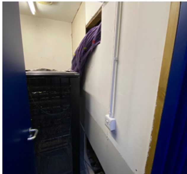
3.3.14 Existing riser cupboard
