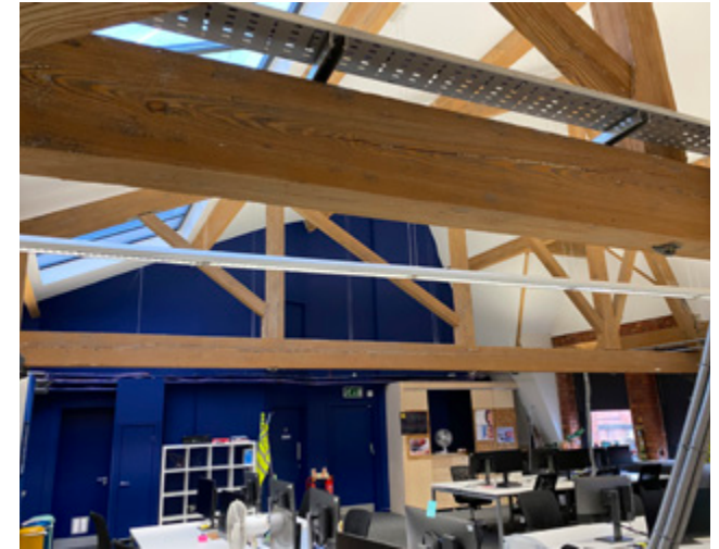
3.3.12 General view to the south interior wall
