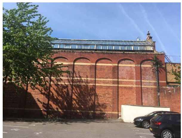
The east elevation of the Females pool, note restrained detailing.
