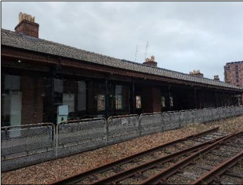
Photograph 3 showing the Station Building
