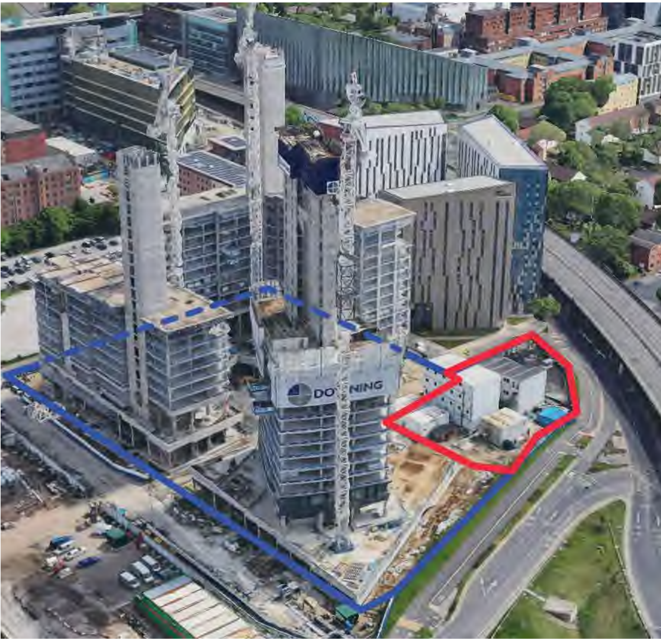
View from the North West, site currently occupied by site cabins for the construction of blocks A, B and D.
