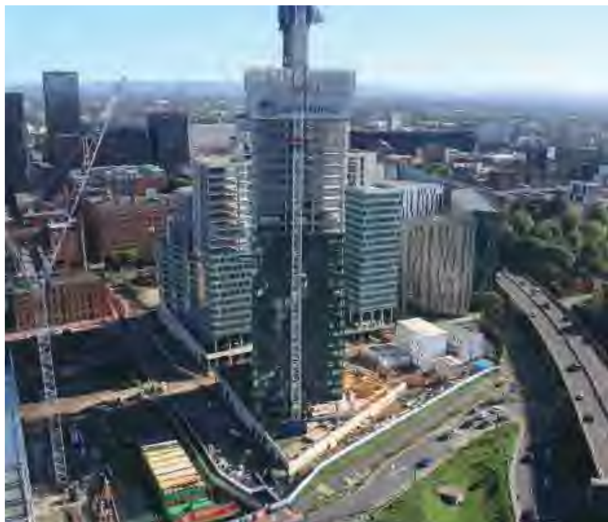
Aerial photo highlighting the current construction on site of blocks A, B and D in the foreground of the image.
