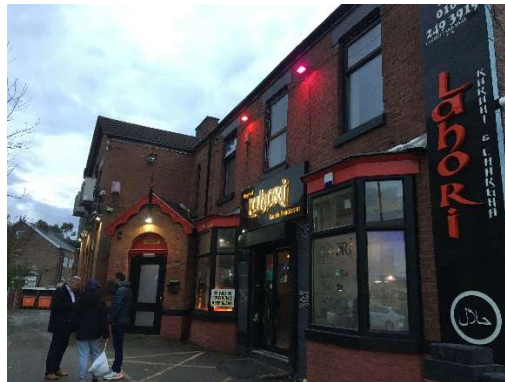
Position of External units of air-conditioning/heating system
