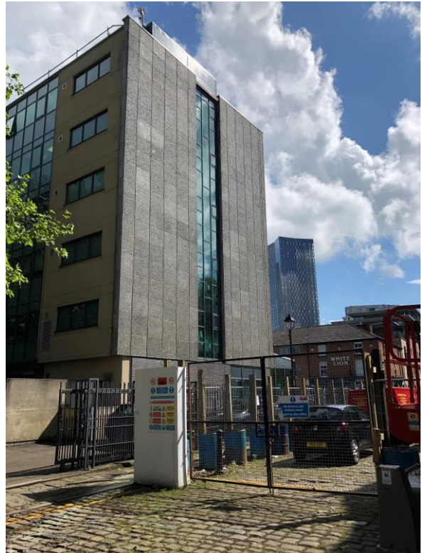
Figure 7: The same view as appeared in October 2023 (Source: SLHA Oct 2023).
