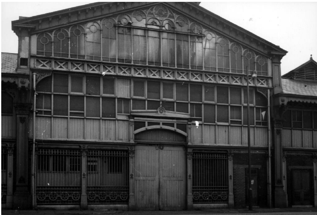
Figure 58: A 1964 view looking at the Lower Byrom Street elevation, showing its dishevelled paintwork/mismatched window repairs and changes (Source: Manchester Archives)
