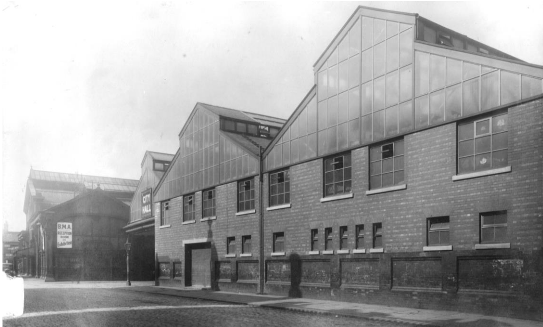
Figure 41: The newly completed City Hall extension (right), known as “New Hall” seen looking south from Byrom Street in c1927 after the extension was constructed upon the original lower walls of the old hay and straw market. The original part of the City Hall, or “Main Hall”, can be seen to the far left. Note that originally the new hall was connected to the main hall via a third, first floor hall/circulation space that spanned across Tonman Street, and was called “Tonman Hall”. (Source: Manchester Archives)
