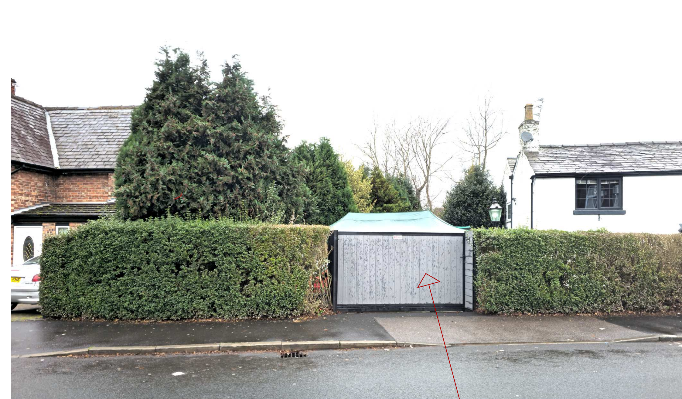
Existing Site Photo
