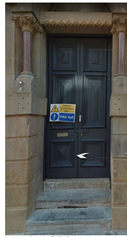
Image of door DG15 to be repaired. Entrances to nos 14 and 16 to be similarly refurbished.
