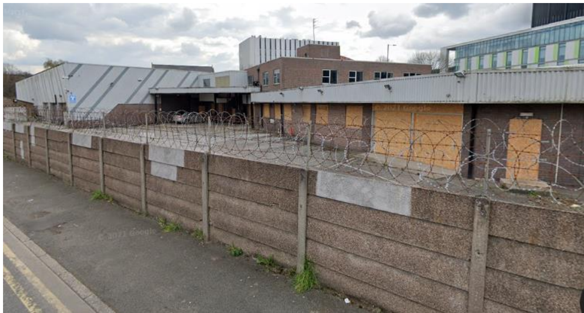
Figure 2.2- Image of existing Site
