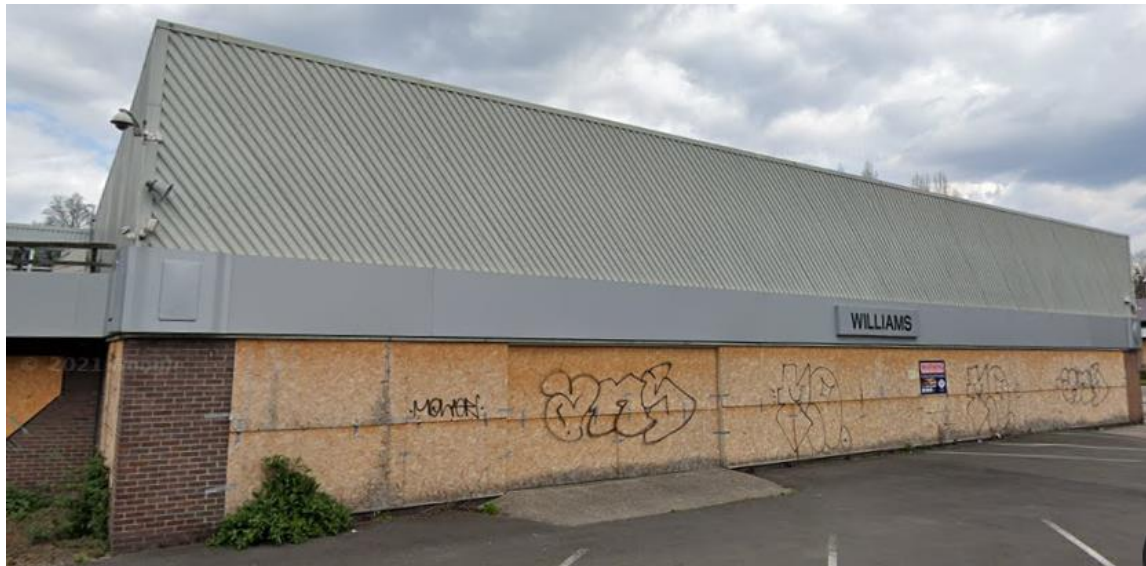
Figure 2.1- Image of existing Site
