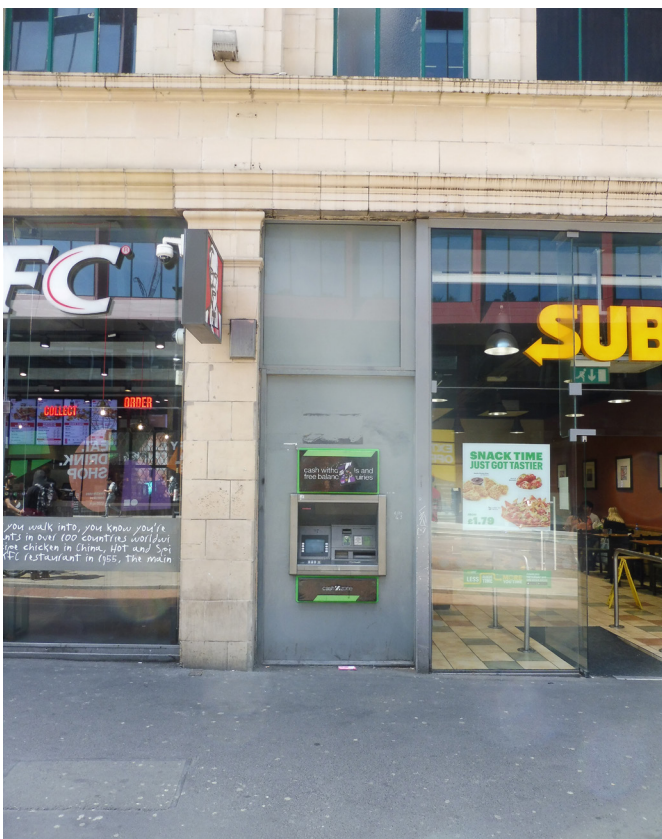
Image 01: 12 Oxford Road - External Facade
