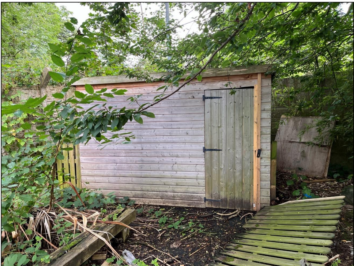
Plate 4 – Timber shed structure at northern site boundary
