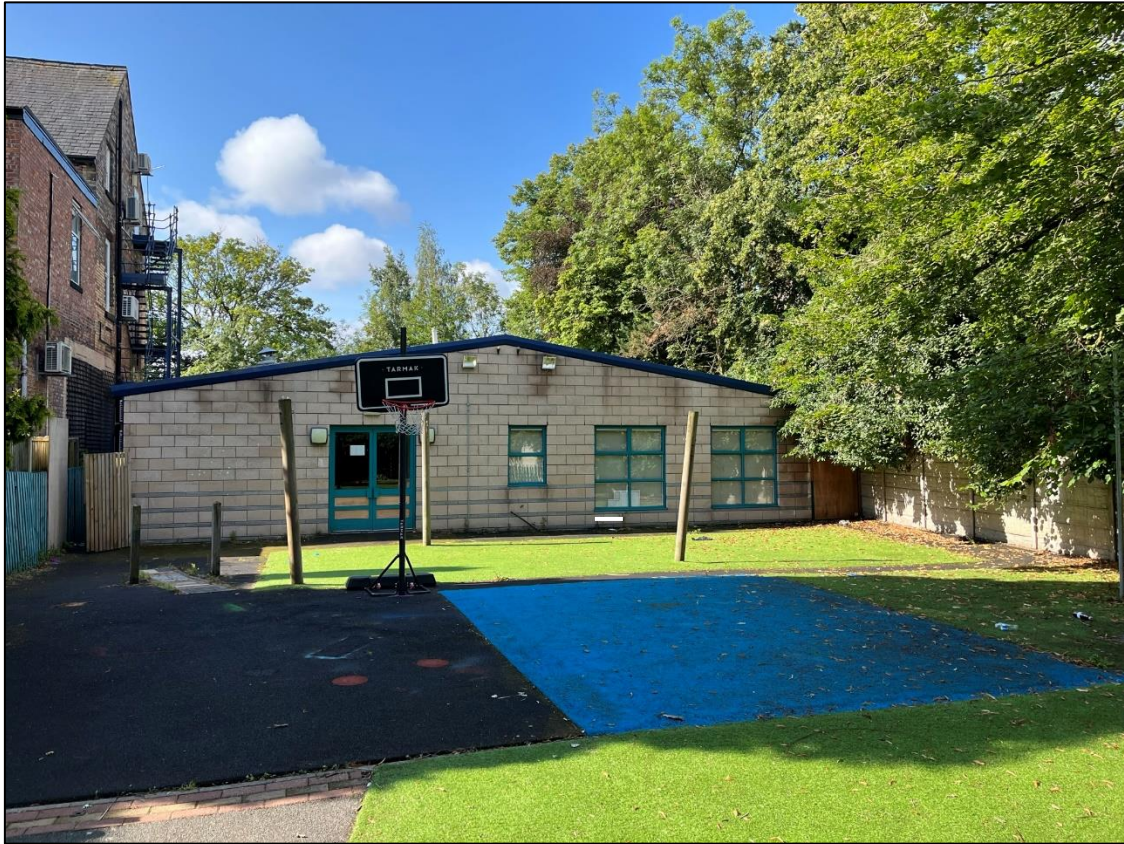
Plate 1 – The northern elevation of the main building, with hardstanding and artificial grass area
