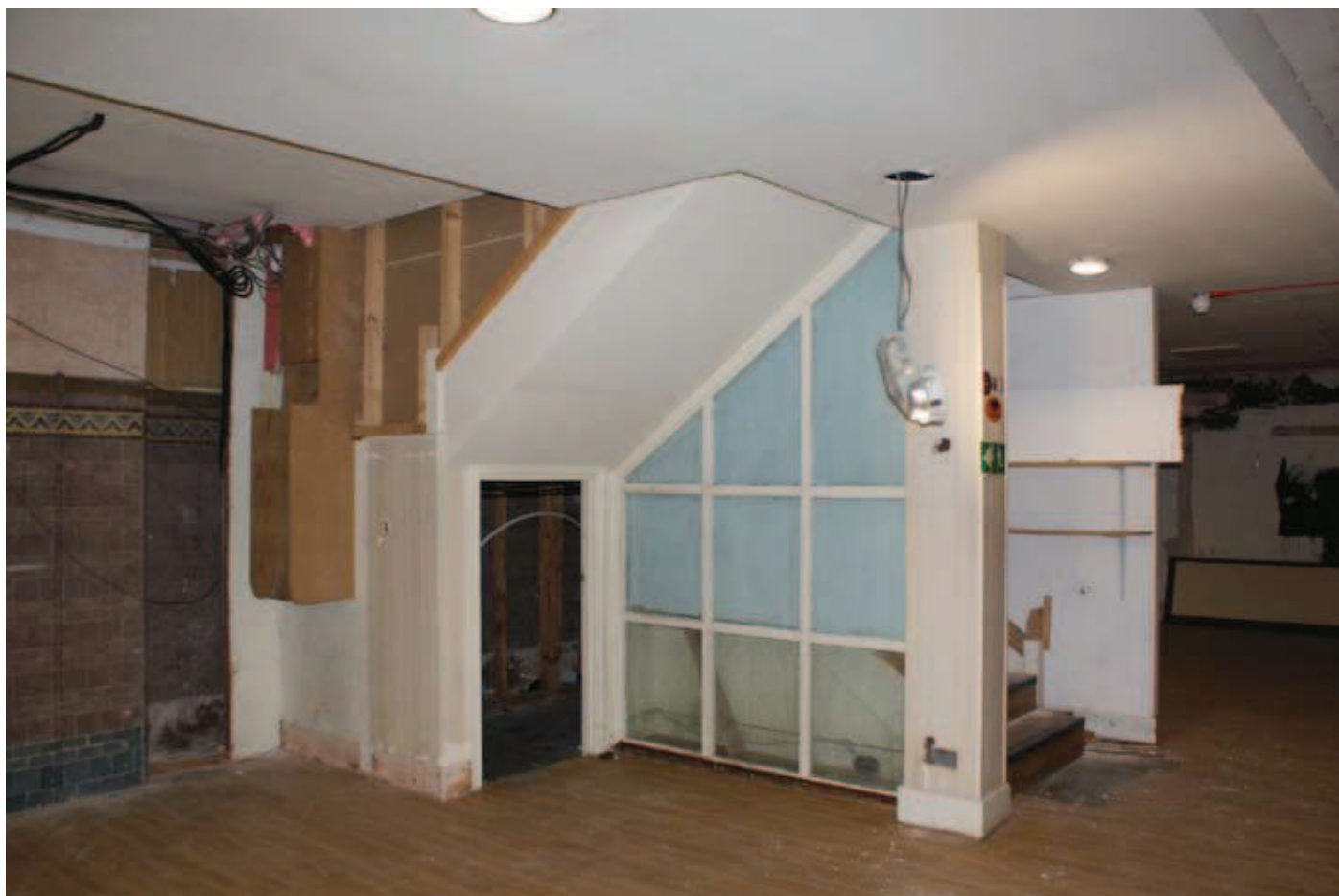
Image of tiling in basement, extending under the current staircase.
