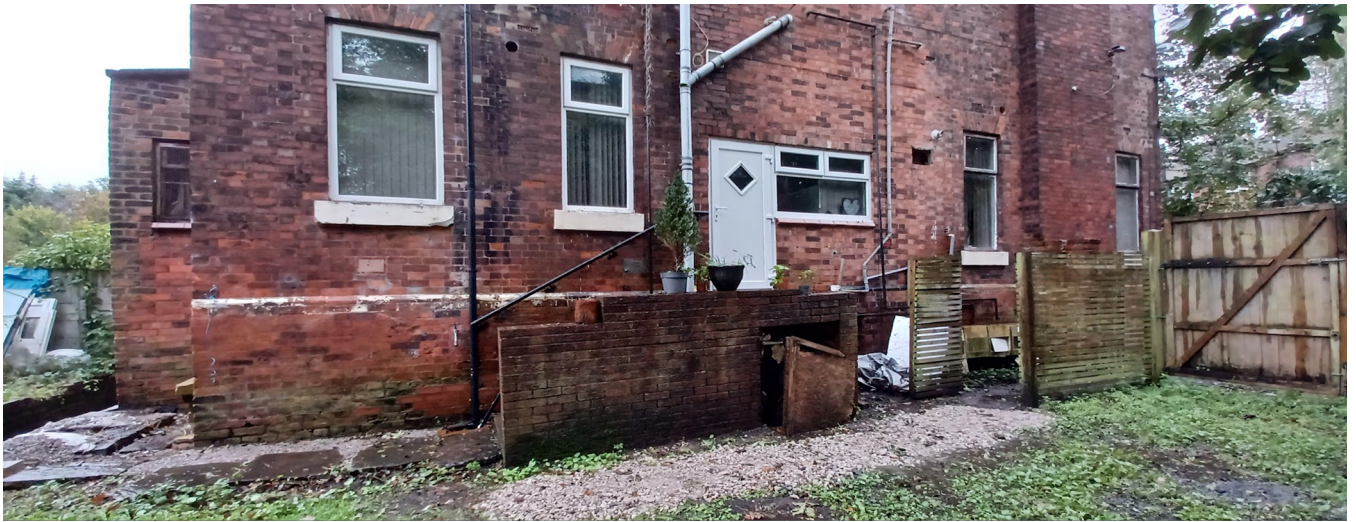
Figure 5. Side of property.
