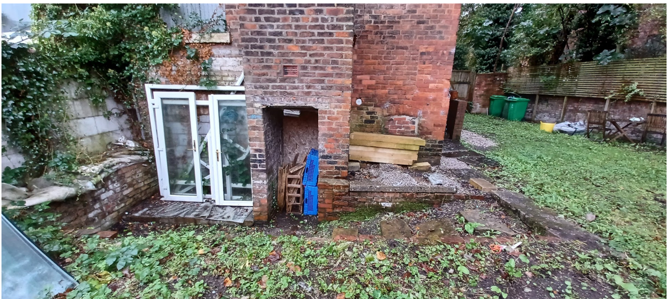
Figure 4. Rear of property.
