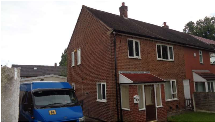
Front Elevation to Application Property.
