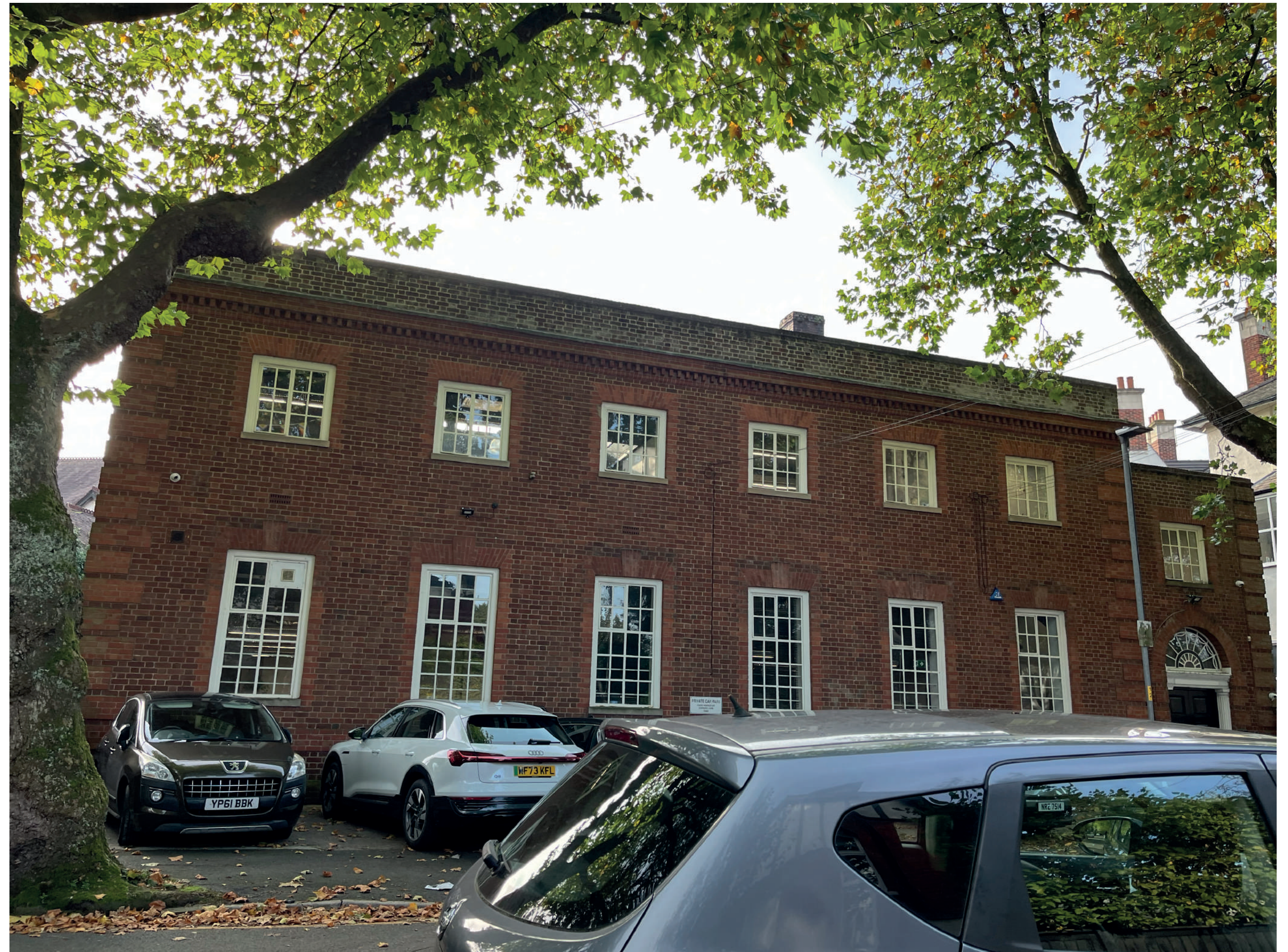
Ballbrook Avenue elevation of Craig House
