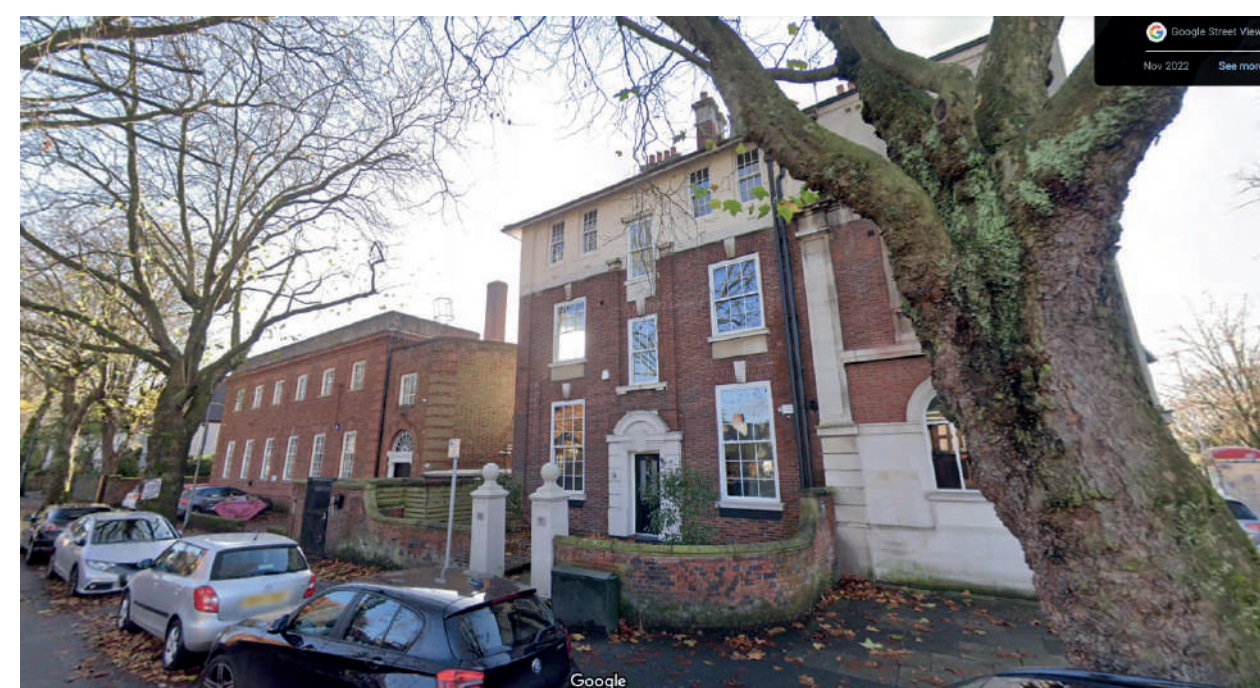
View of the municipal building block from the end of Ballbrook Avenue. Bank building to the right, Craig House to the left.
