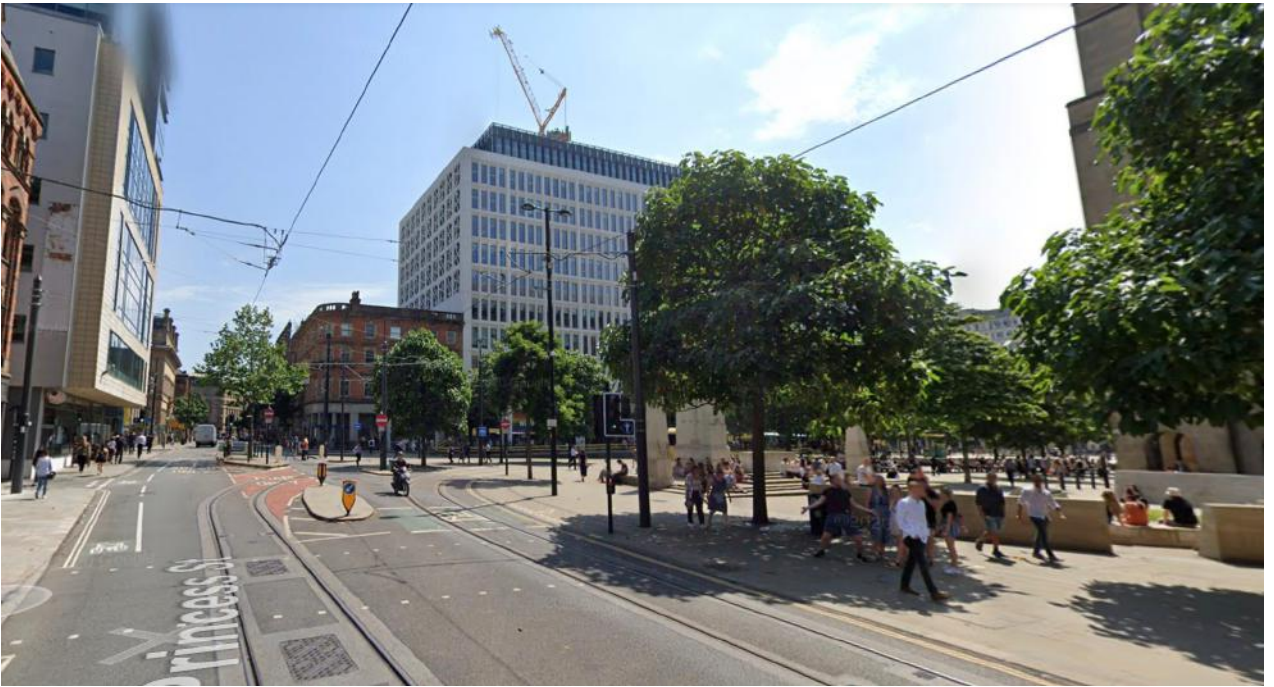
Image 4: Contemporary views of site, looking towards Peter's Square with Manchester Town Hall extension to right and site to far left.
