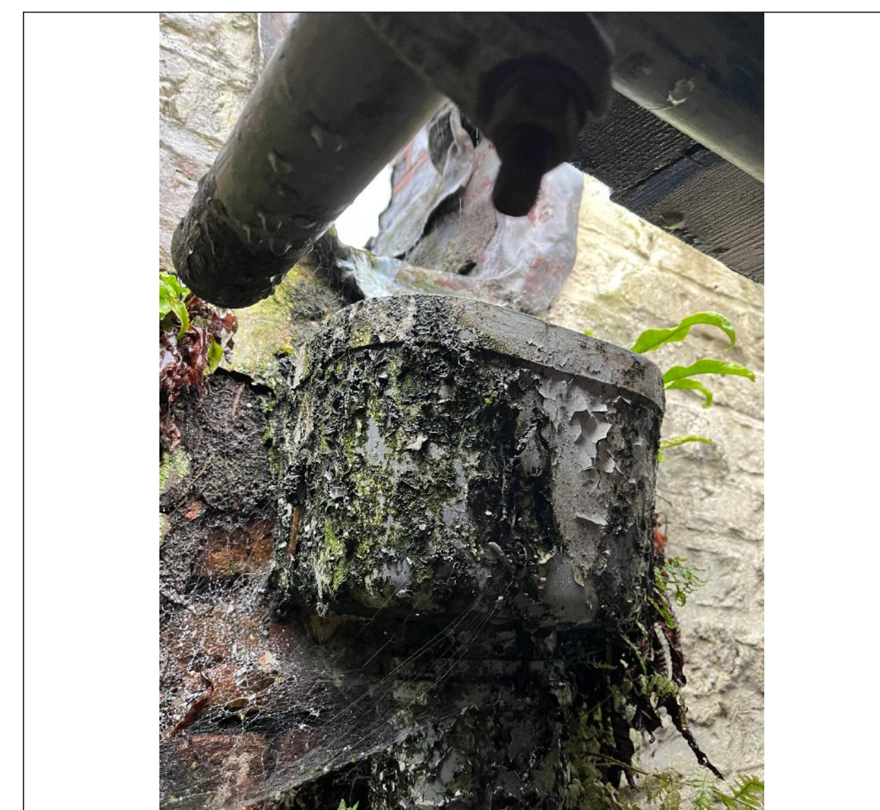
Image 17: Detail of plastic rainwater goods to lightwell.
