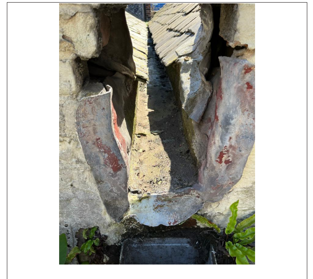
Images 12,13: Top: Roof detail. Bottom: Detail of existing gutter and slate junction.
