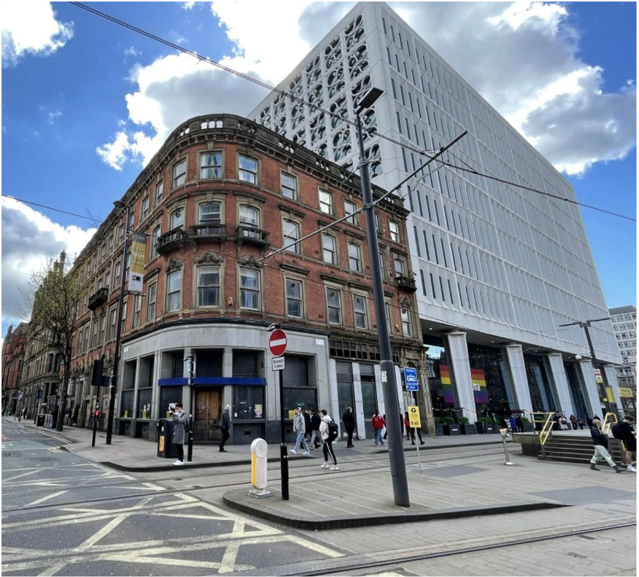
Image 3: Contemporary photograph of 77-79 Mosley Street, with the modern block of 2 St. Peter's Square to the right.
