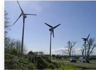
Wind Turbine Installation
