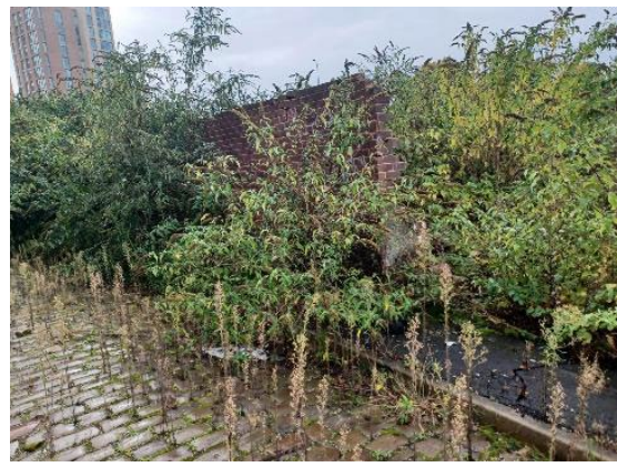
Photograph 8: brick wall to the south of cobbled road
