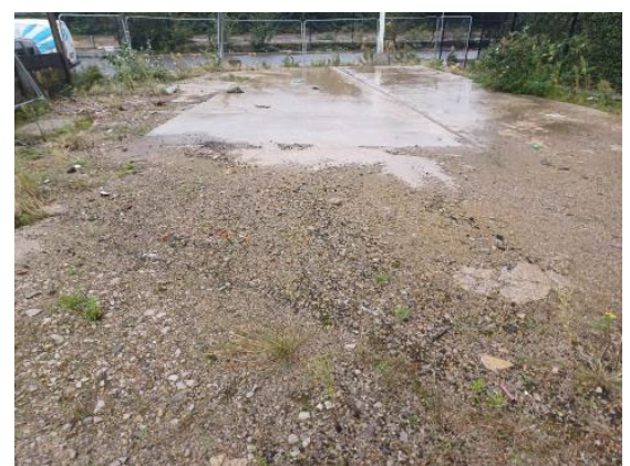
Photograph 6: concrete slab and gravel surfacing in the north
