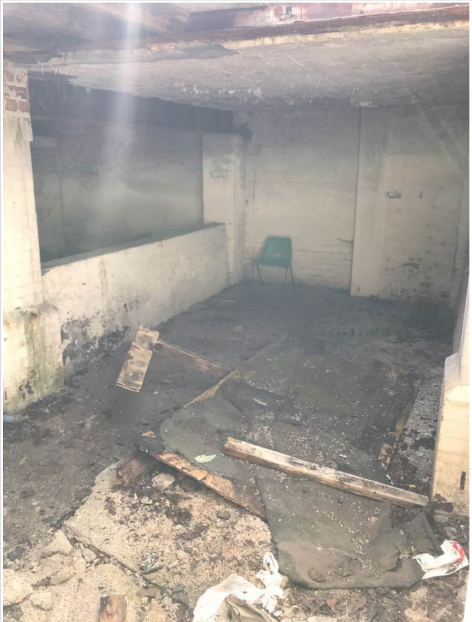
View from front elevation to rear (west) wall :- Brick buttresses form part of west wall which forms external wall to shops
