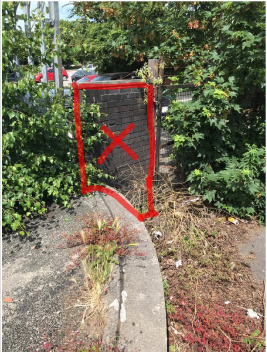
3/ Remove external brick wall located by boundary gate (1365 x 1880mm)
