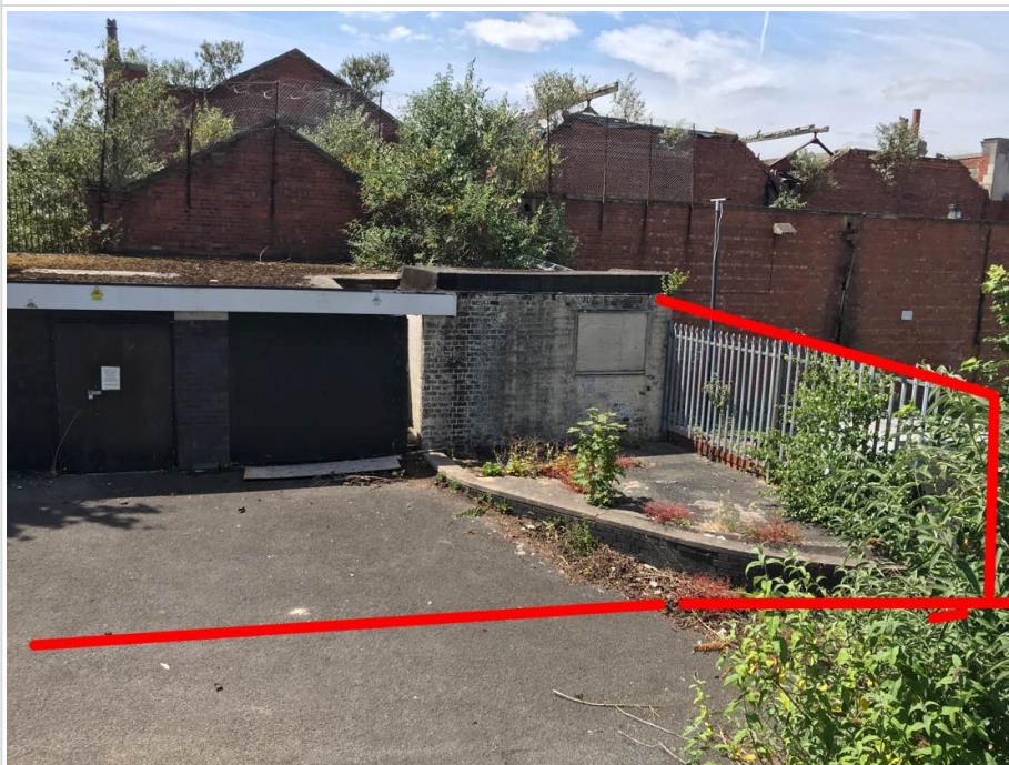
Timber Hoarding across 14.5m front elevation with 7m return as shown
