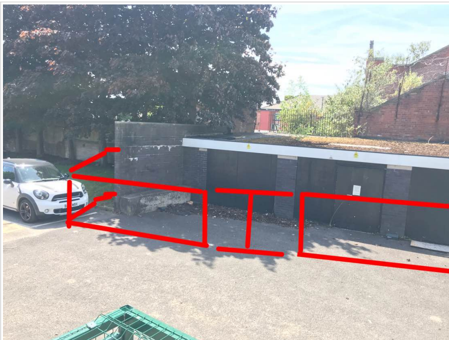
Timber Hoarding - with gated access
