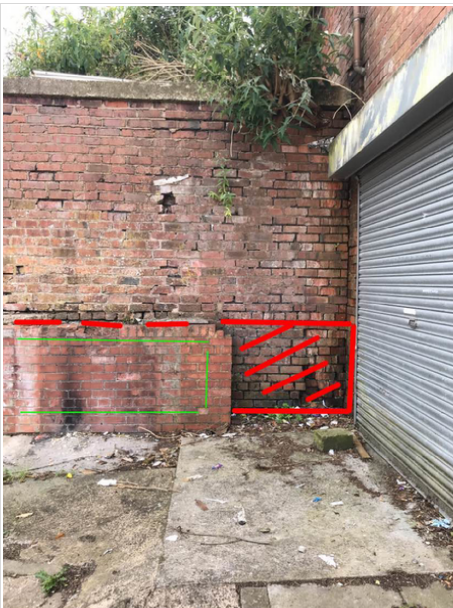
North wall - Rebuild structural wall as part of existing support to proposed vehicle parking bays above.
