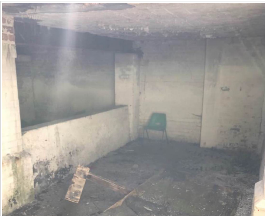
West wall , internal view :- 14.8m x 2.2m
