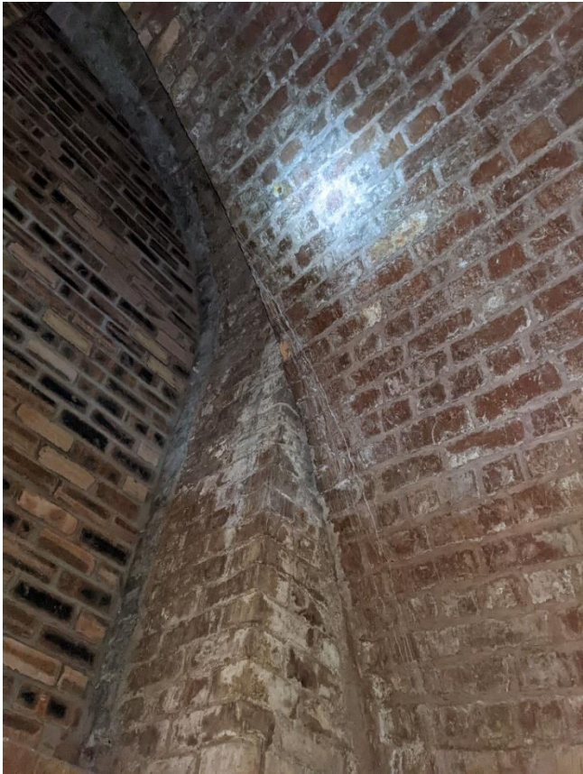
Figure 2-7 Typical condition of viaduct arches
