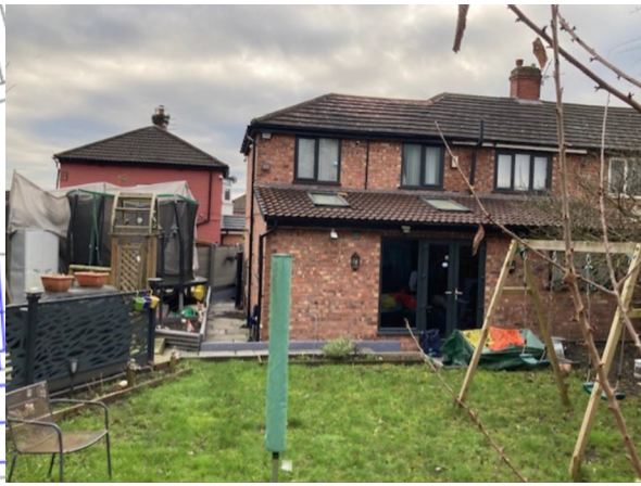
View of the rear of the property
