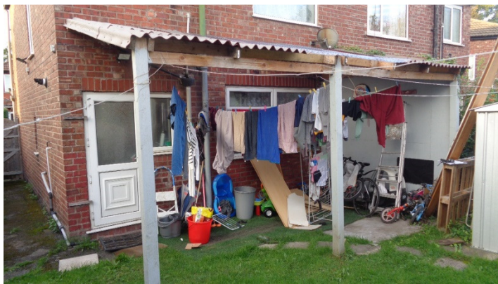
Rear Elevation to Application Property.
