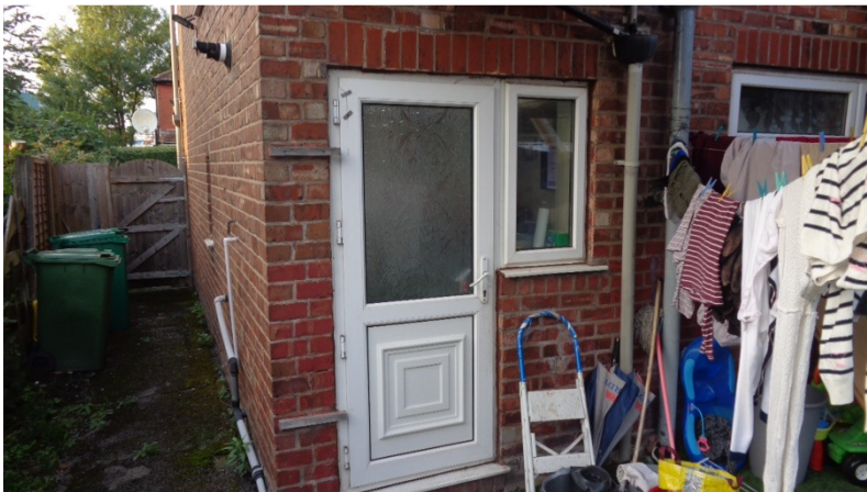
Rear Elevation of Application Property.
