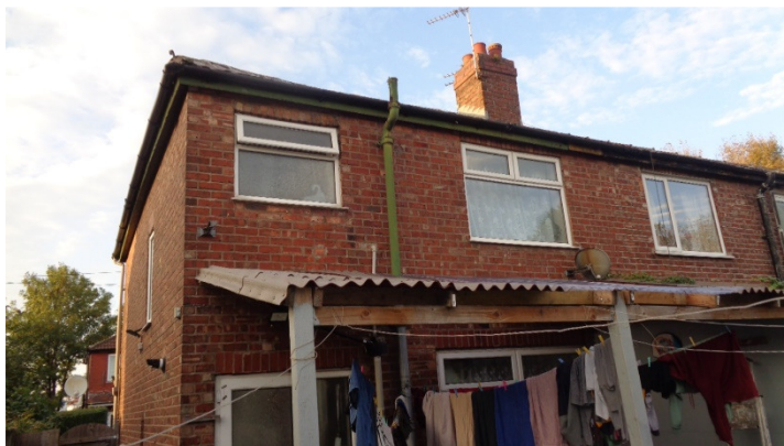
Rear Elevation to Application Property.
