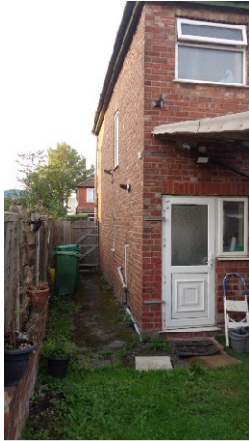
Gable Elevation of Application Property.
