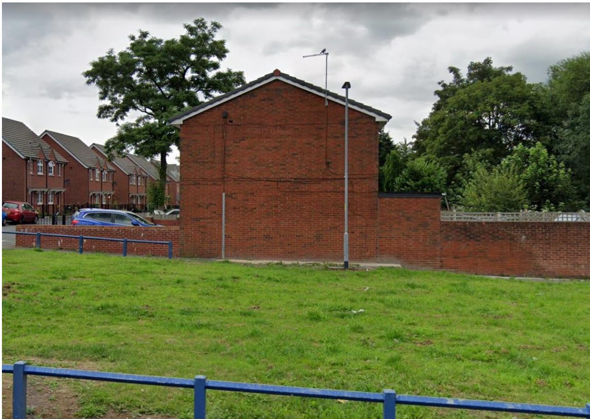
Figure 8.2 – Existing Openreach infrastructure as indicated on Google street view
