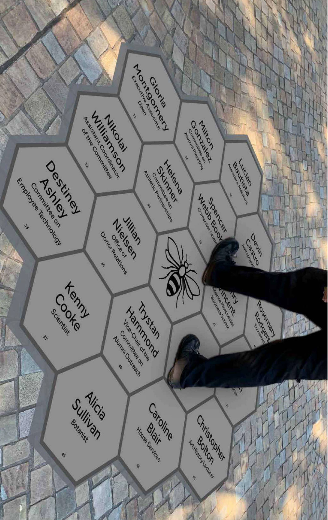
SAMPLE OF PROPOSED KILKENNY BLUE FLAMED LASER ETCHED PAVERS; PHOTO OF STONE WET
