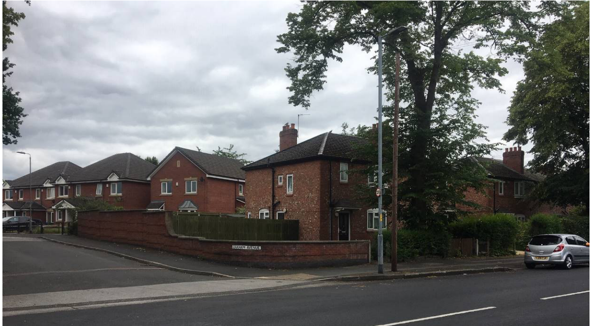
View to site from Mauldeth Road West
