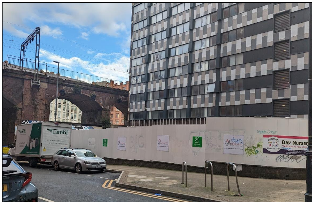
Plate 2 View of site from York Street, October 2023
