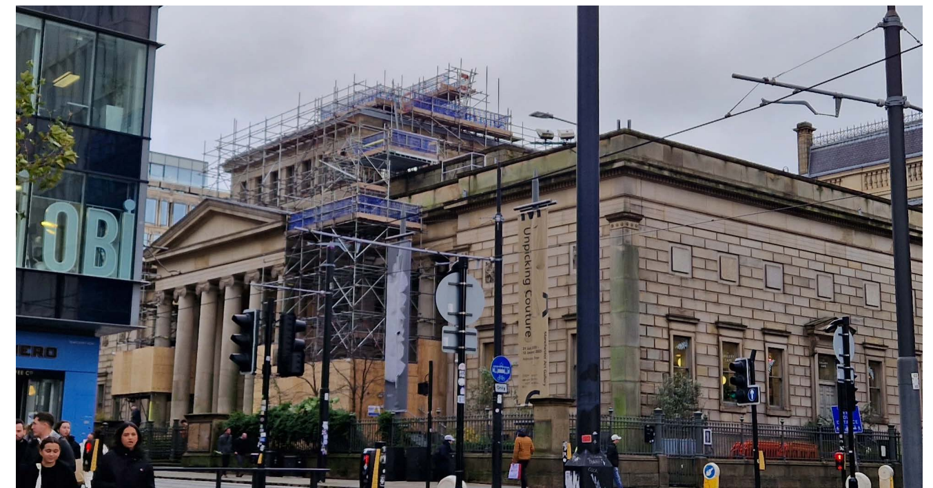
Figure 17 Roof Lantern Inspection Scaffold, viewed from St Peter's Square
