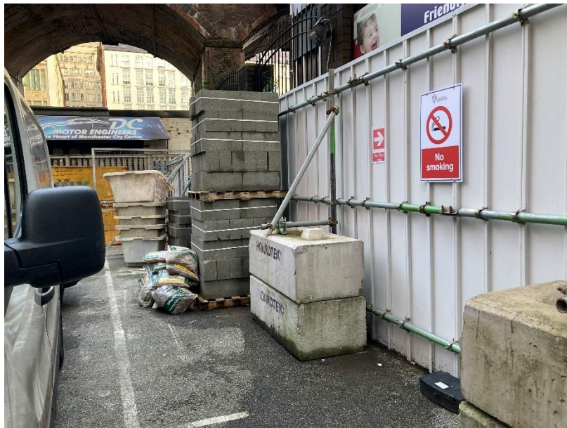
PLATE 1 SHOWING AREA OF HARDSTANDING
