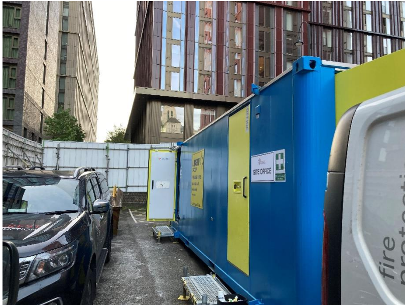
PLATE 2 SHOWING THE ON-SITE BUILDING
