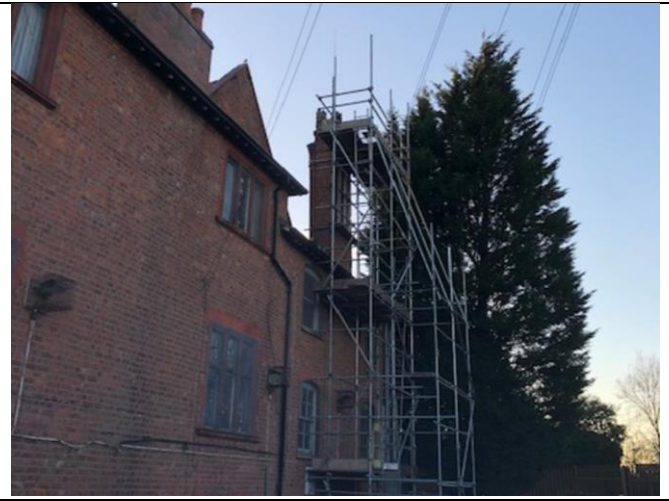
Chimney in Proposal located behind Scaffold.
