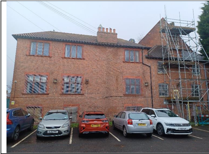
Chimney in Proposal located behind Scaffold.
