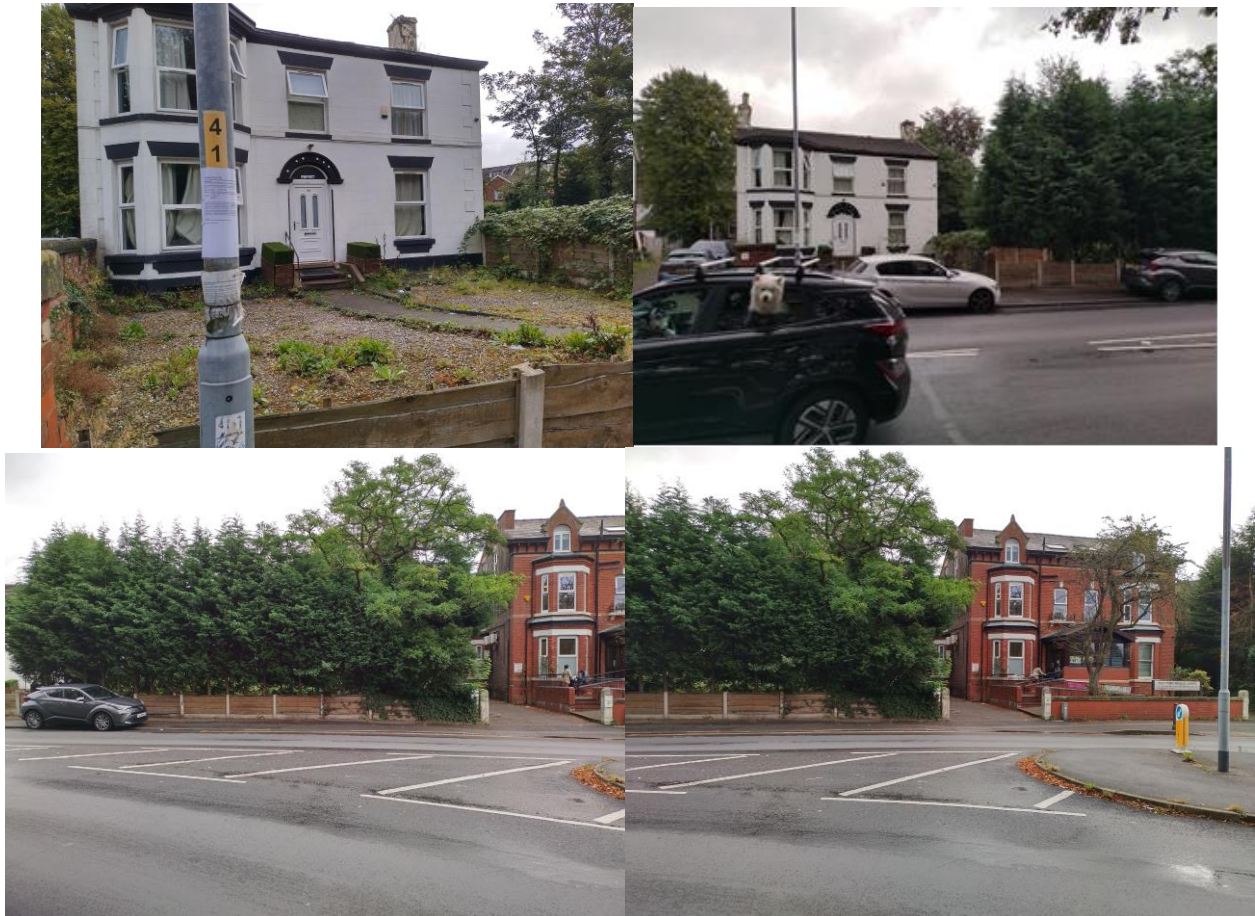
Fig.2 – 161 Slade Lane and the application site
