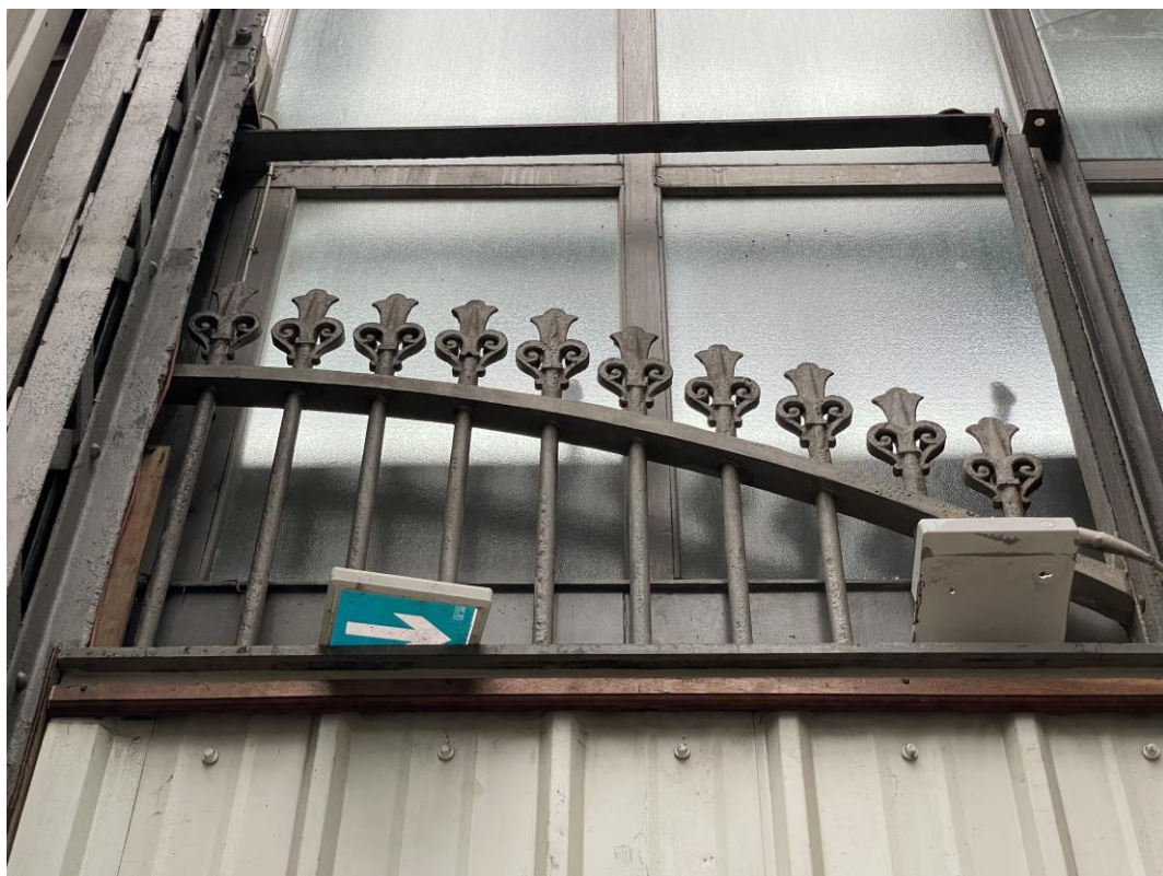
Figure 91: A closeup of the top of the concealed northernmost gate.
