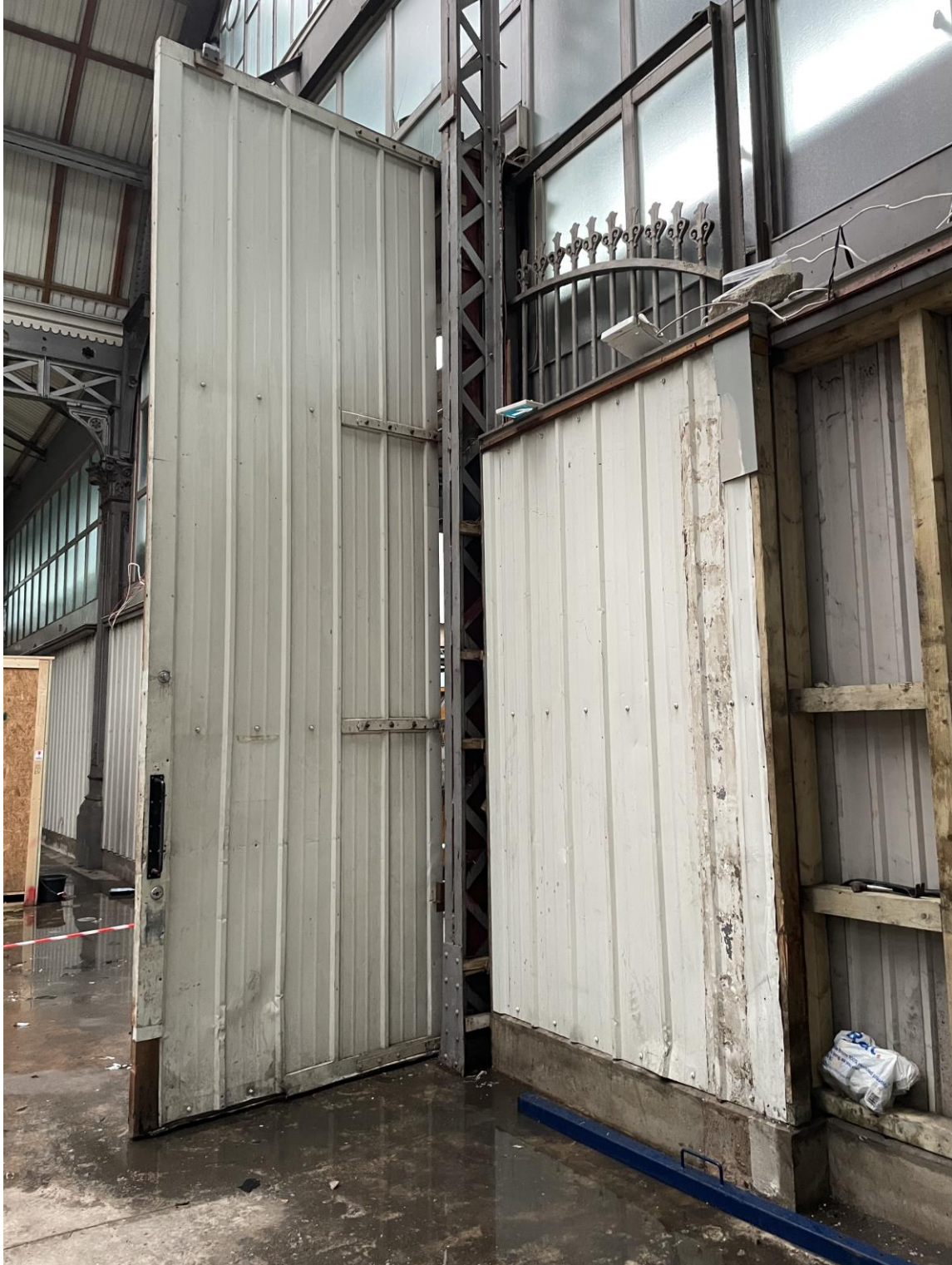
Figure 89: The western entrance from Barton Street, showing the modern 1980s corrugated metal doors, which conceal the only surviving pair of original cast iron gates within the building.
