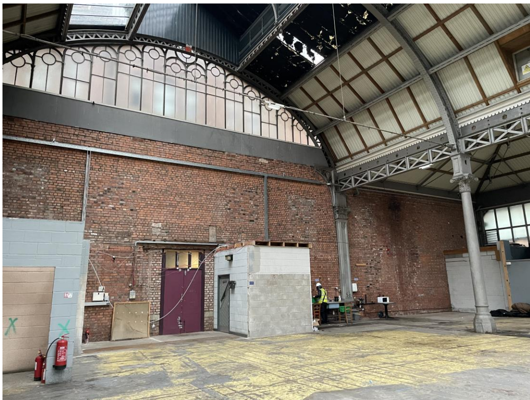
Figure 83: The 1894 east elevation.
