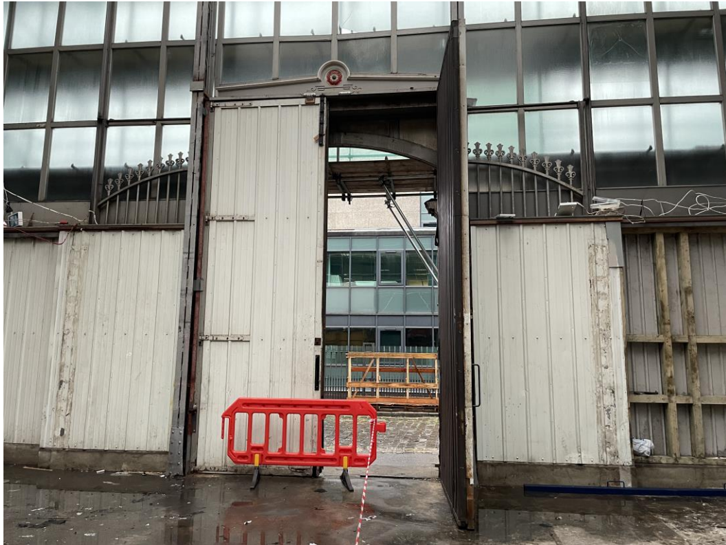
Figure 90: The west entrance showing the two original gates protruding to either side of the modern 1980s doors.
