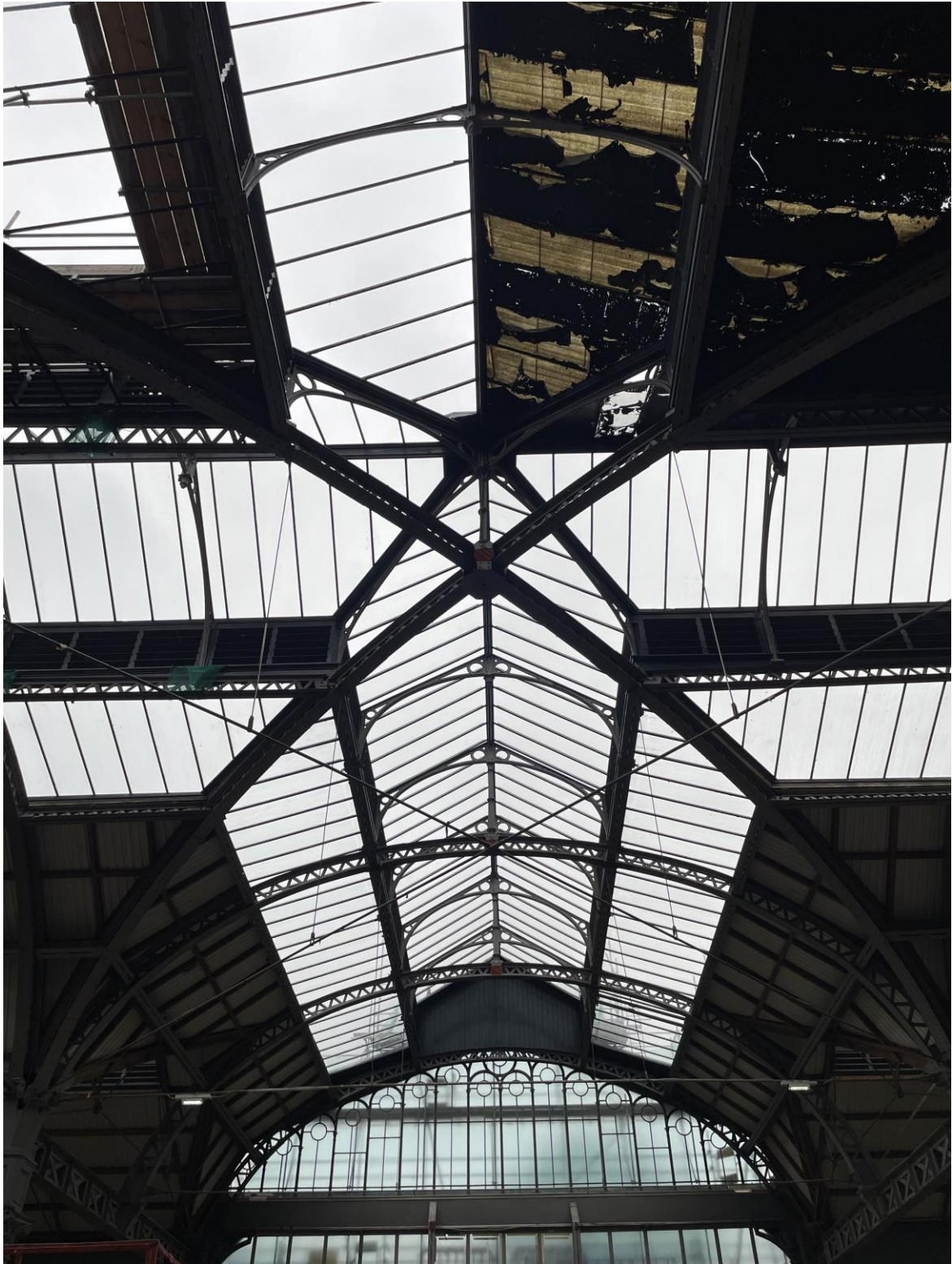
Figure 97: A view looking north up at the roof structure.
