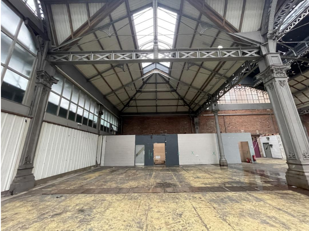
Figure 80: Looking east along the northern side of the building. The brick eastern wall was constructed in 1894 as part of the formation of the auction room.
