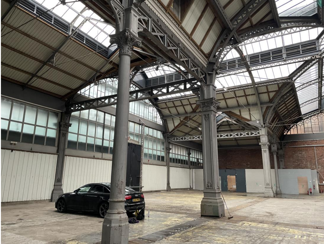
Figure 78: Looking north-east along the north, Tonman Street elevation.
