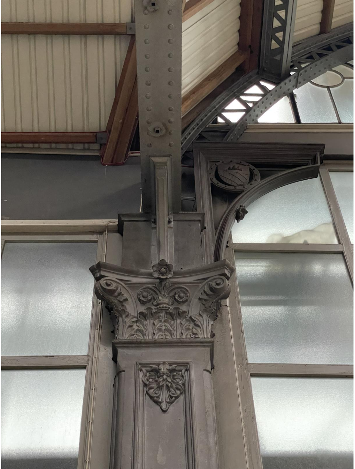
Figure 95: Detail of one of the Corinthian capitals to the northern external wall.
