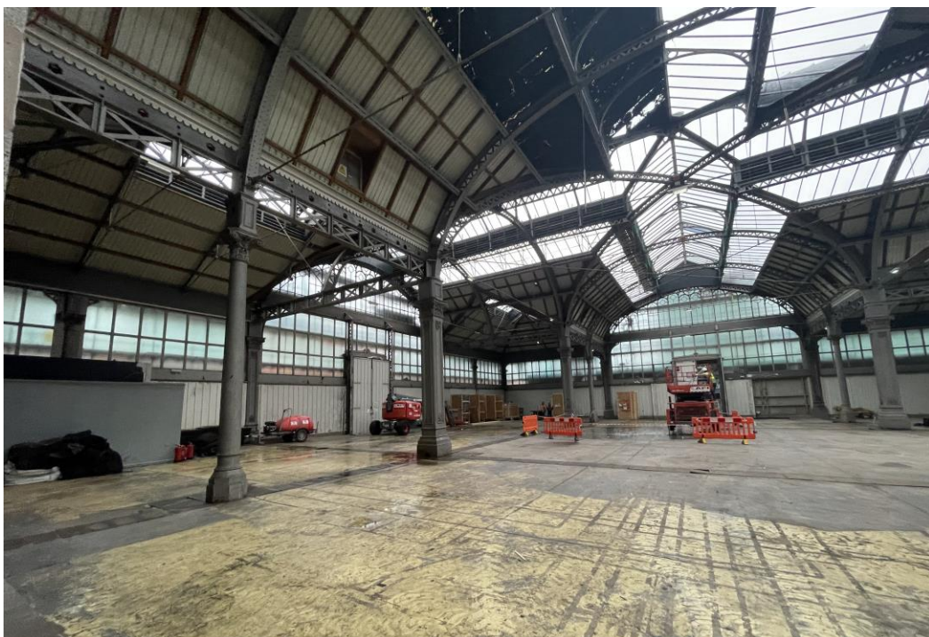
Figure 88: Looking west through the market from the east elevation.
