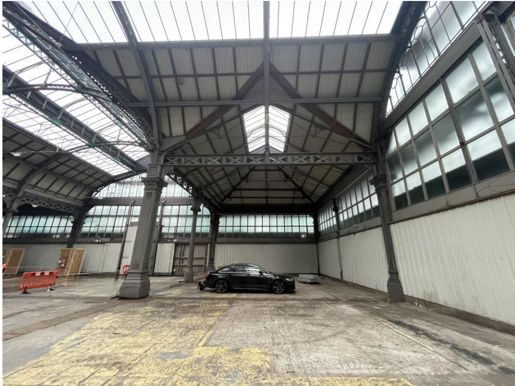
Figure 82: Looking west along the north elevation towards Barton Street.
