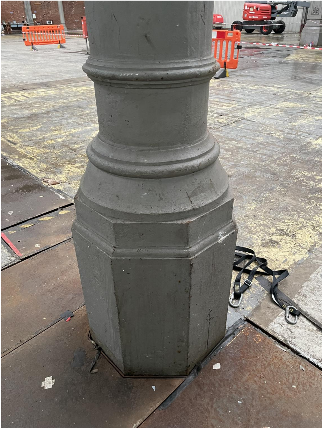
Figure 92: Detail of one of the original cast iron column bases.
