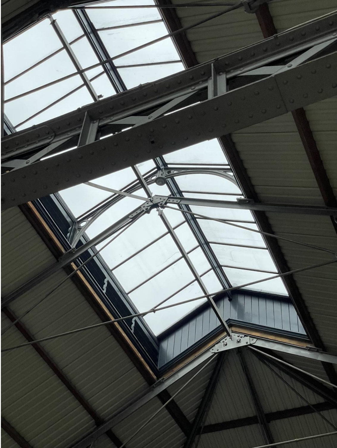
Figure 84: Detail looking up at the south-east corner lantern.
