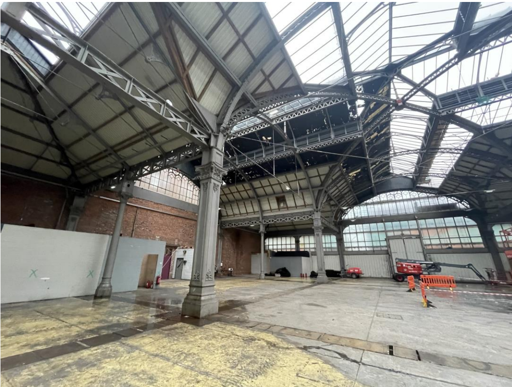
Figure 81: Looking south-east from the north elevation.
