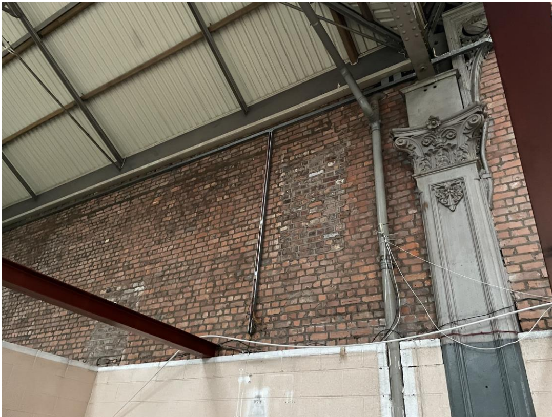
Figure 86: Detail of the interface between the original 1870s cast iron external column and the 1894 brick infill to the east elevation.
