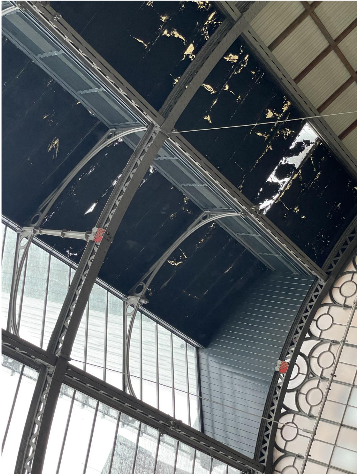
Figure 96: A view looking up at the raised central roof structure towards the east elevation.
