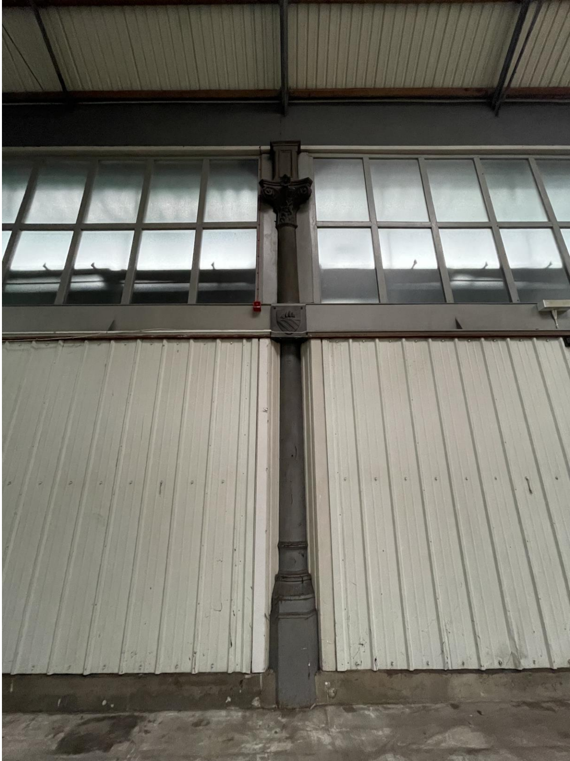
Figure 94: An example of one of the external columns to the north elevation.
