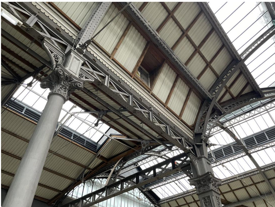
Figure 79: Detail of the cast and wrought iron columns and roof structure to the north-east corner.
