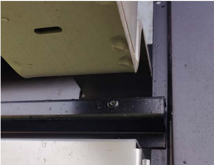
Flashing fixing removed from front face
