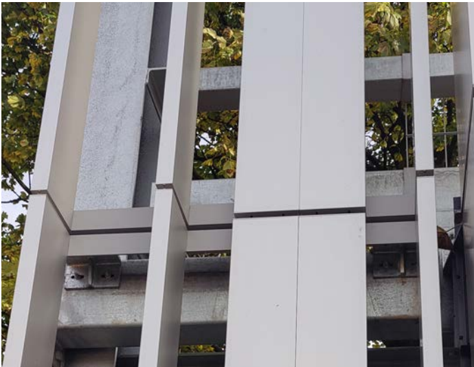
25mm gap between fins
