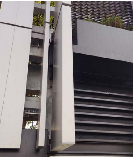
Large fin brackets to be PPC to match the anodised fin
