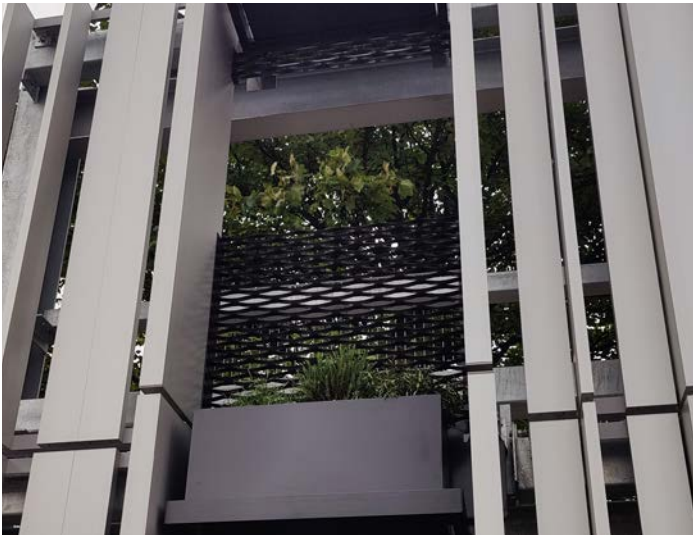
Mesh aperture size to be reduced
