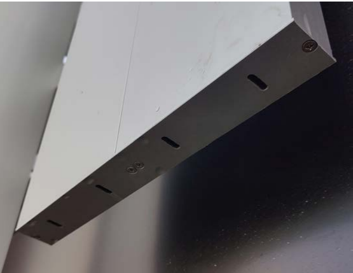
Countersunk screws to underside off small fins
