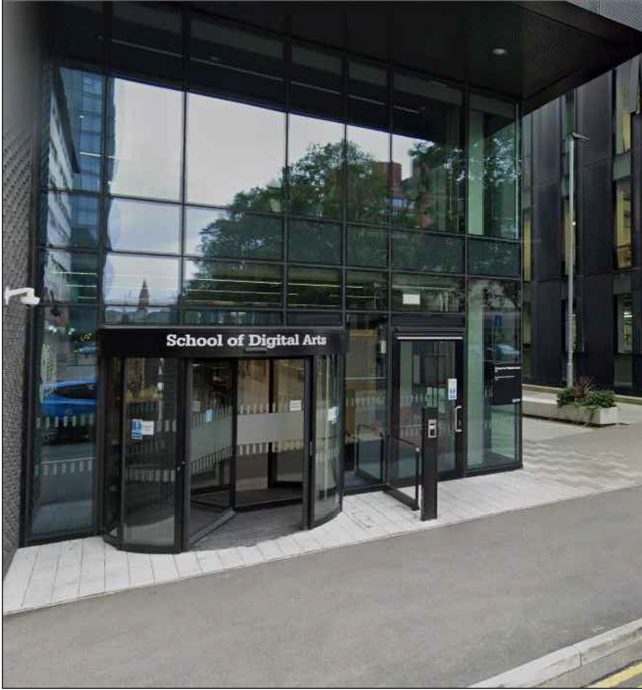
New sign installed
