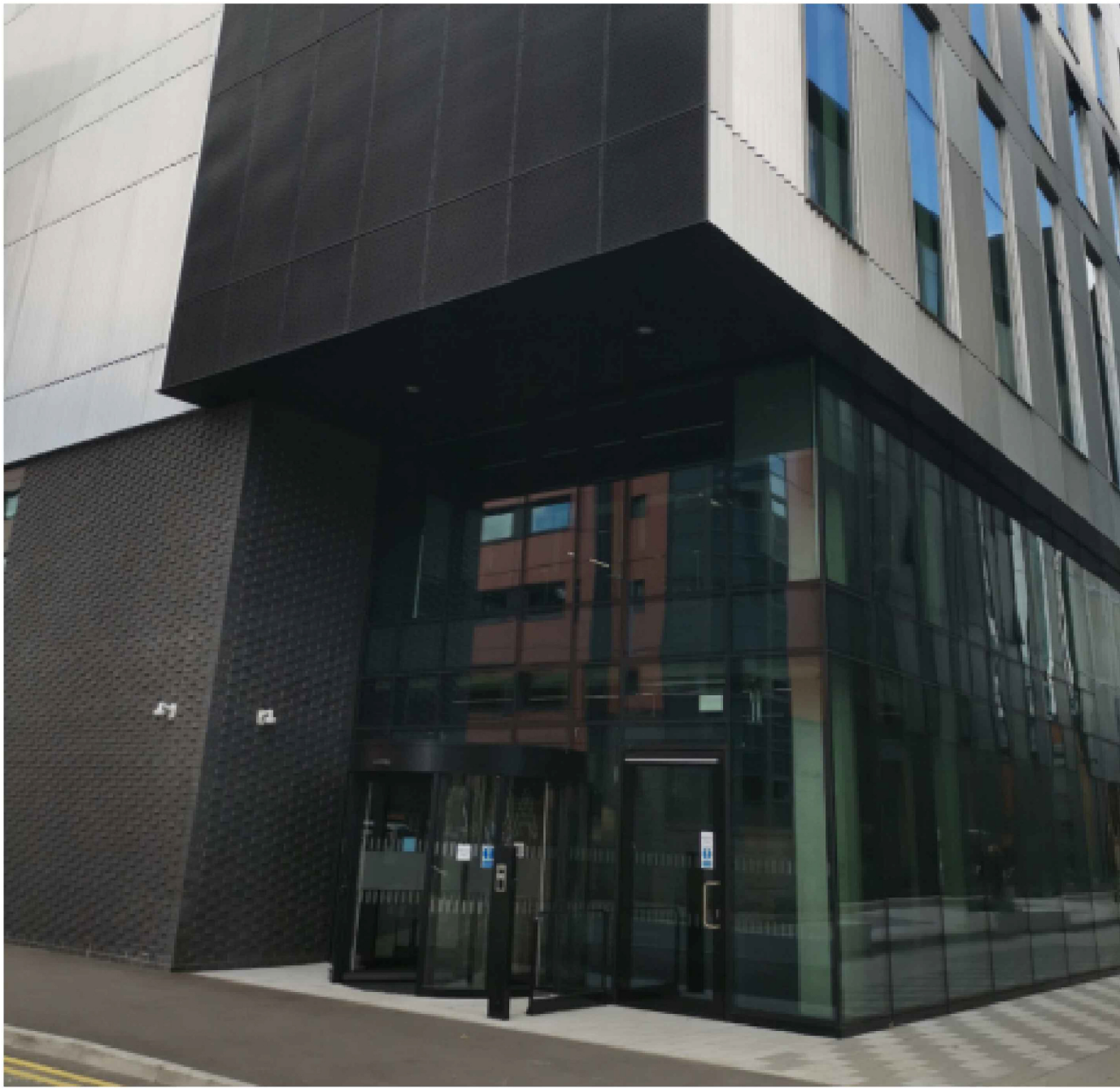
Replaced no sign
