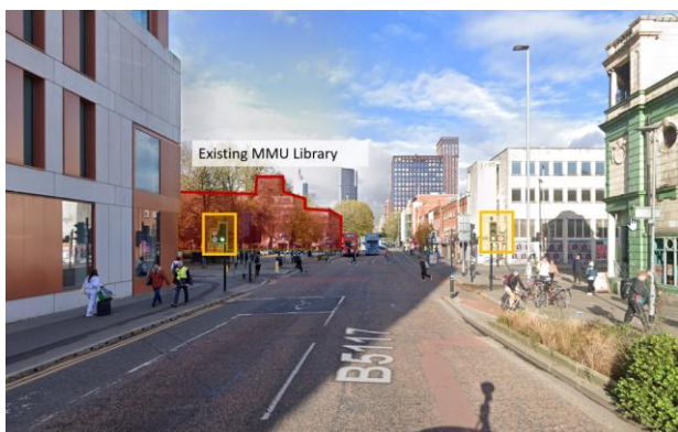
Figure 0-1 View from Traffic light 1 travelling North, existing building
