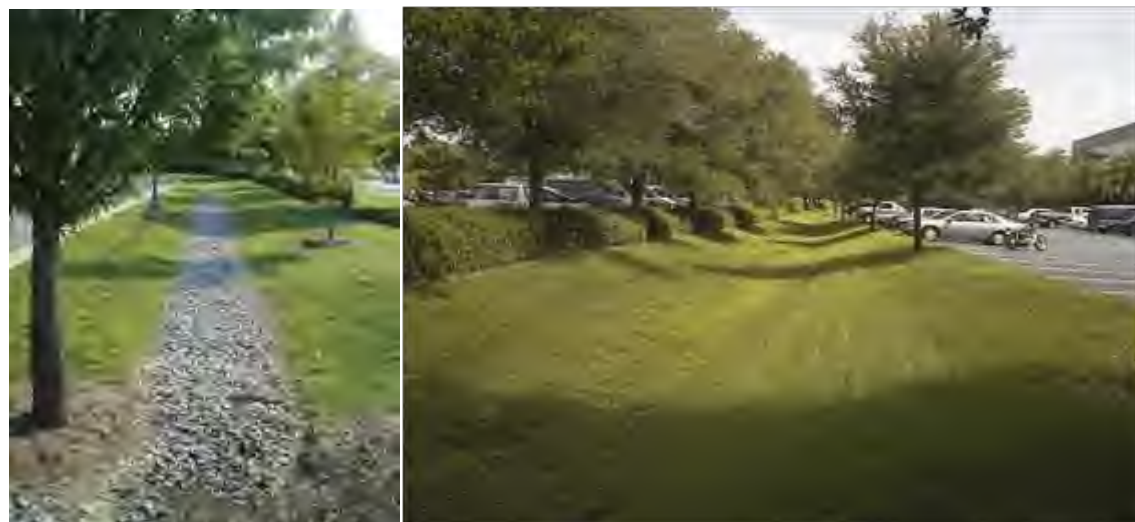
Figure 7-2 Infiltration Trench Example (Left); Swale Example (Right)
