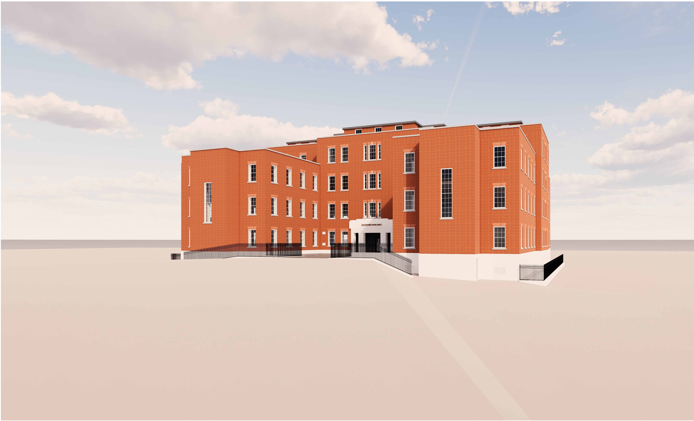
02 - Existing view of the Zochonis Building from Brunswick Street
