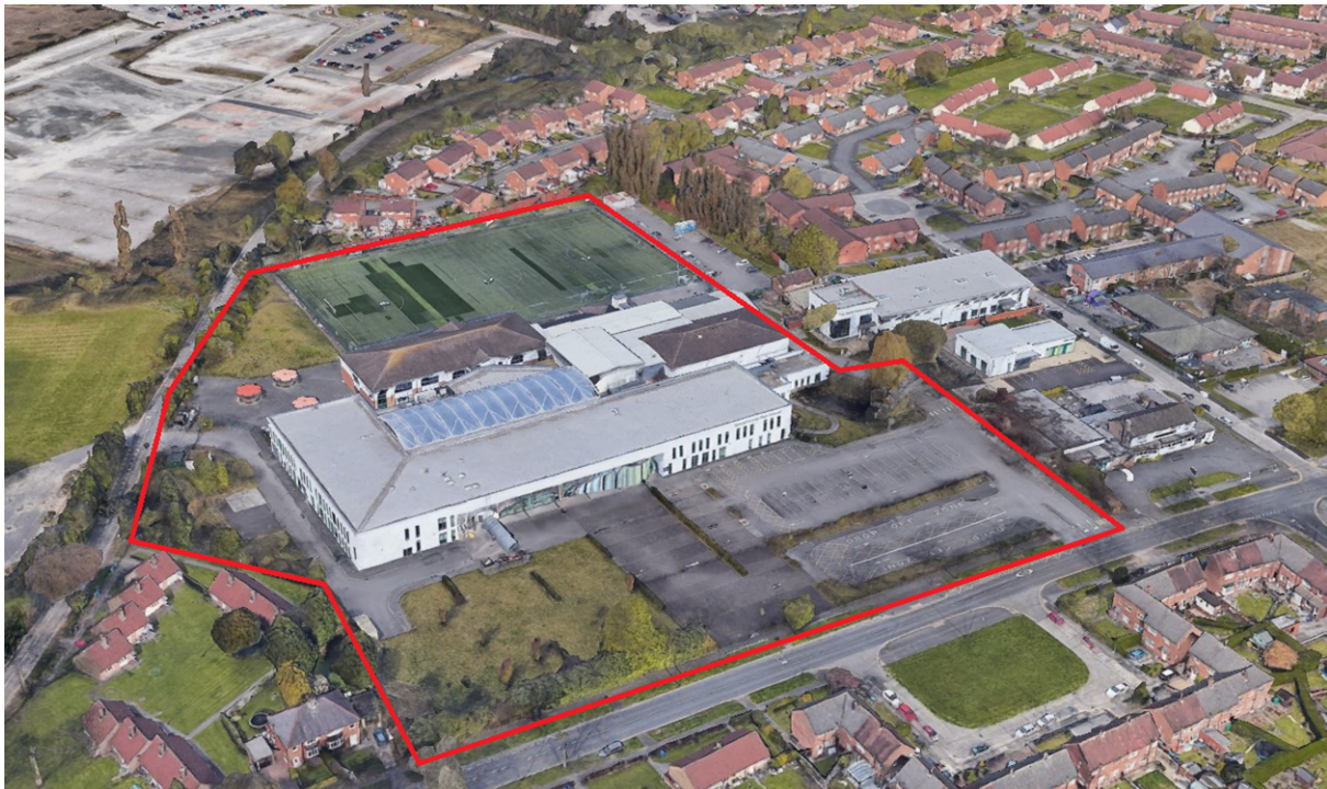
Existing School Site with school buildings located centrally across the site
