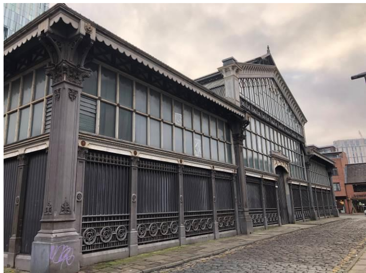
Figure 66: The west elevation on Barton Street, showing the only examples of surviving original cast iron railings to the bottom parts.
