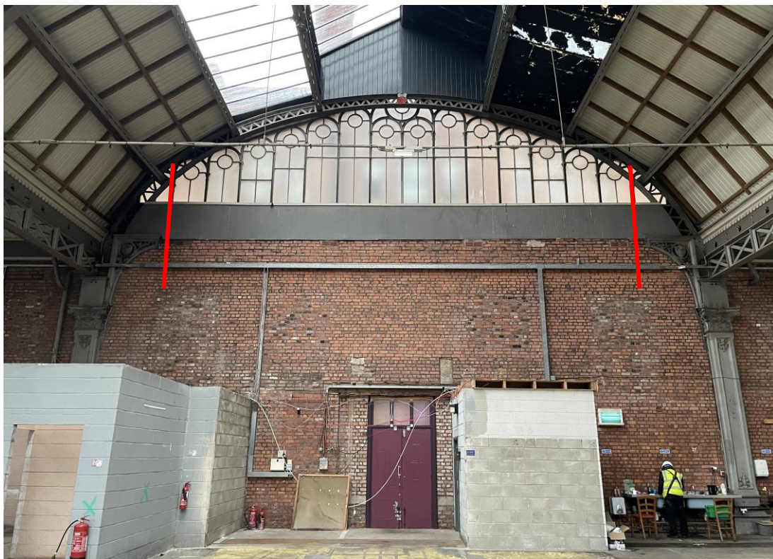
Figure 24: The same view as seen from ground floor level in January 2024. The red lines denote the original sides of the auction room as seen in Figure 23 above. (Source: SLHA 2024).
