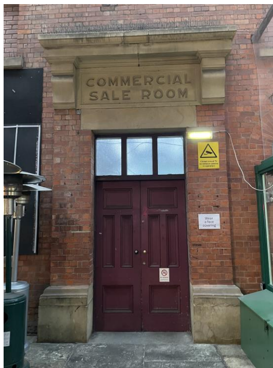
Figure 72: The 1894 Commercial Sale Room entrance which led up originally to the first floor auction room, with viewing sample rooms below.
