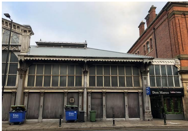
Figure 62: The eastern section of the south elevation, showing the matching link that connects the market building with the former library building (right) across a former market alley.
