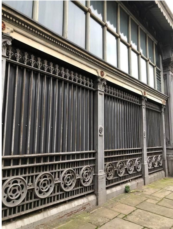
Figure 68: The southern section of the west elevation on Barton Street, showing the only examples of surviving original cast iron railings to the bottom parts.
