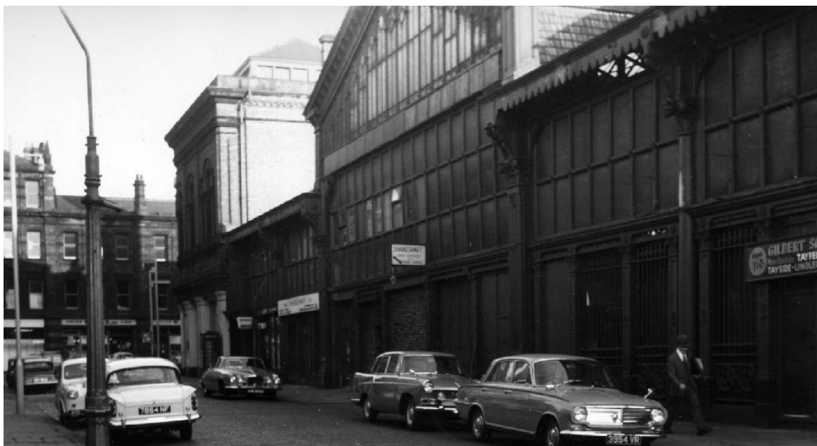
Figure 44: A view looking east from the end of Tonman Street towards Deansgate in 1965. (Source: Manchester Archives)
