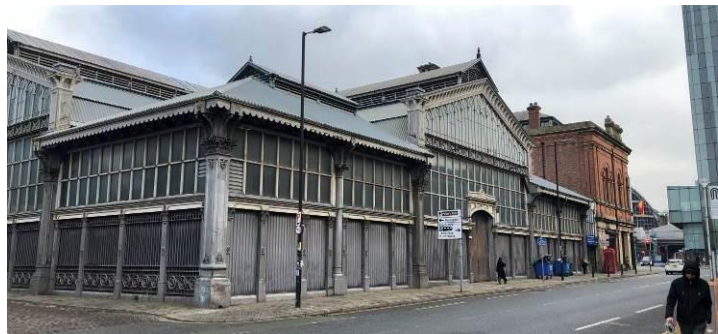
Figure 59: The south elevation (right) and west elevation (left).
