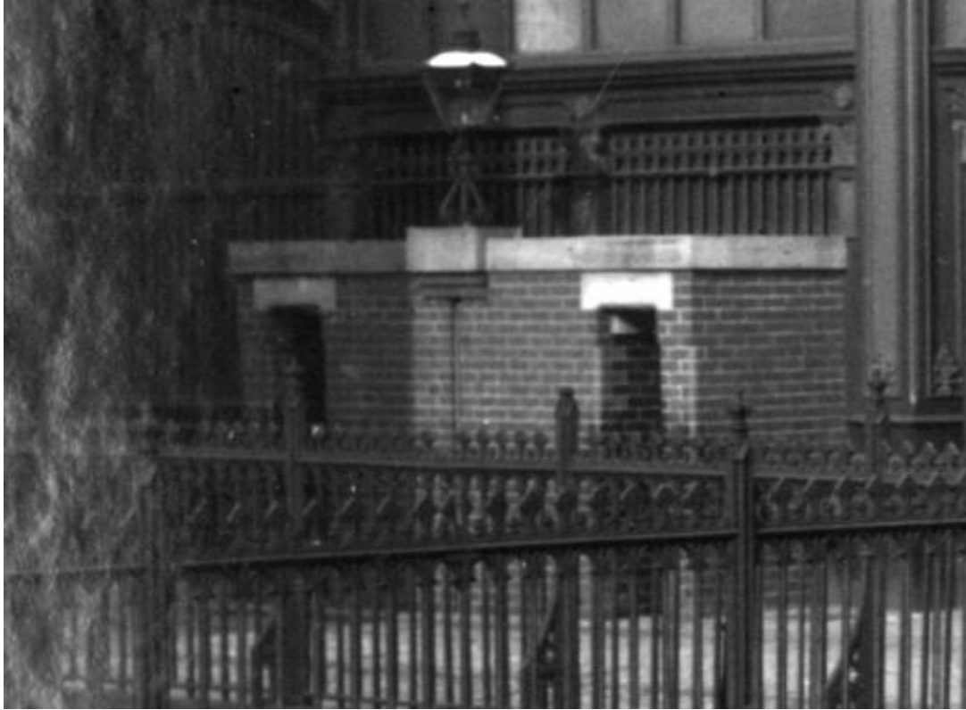
Figure 32: View of the 1881 (or before) men's urinals to the western elevation, which would have, presumably, been utilised by market traders. (Source: Manchester Archives).
