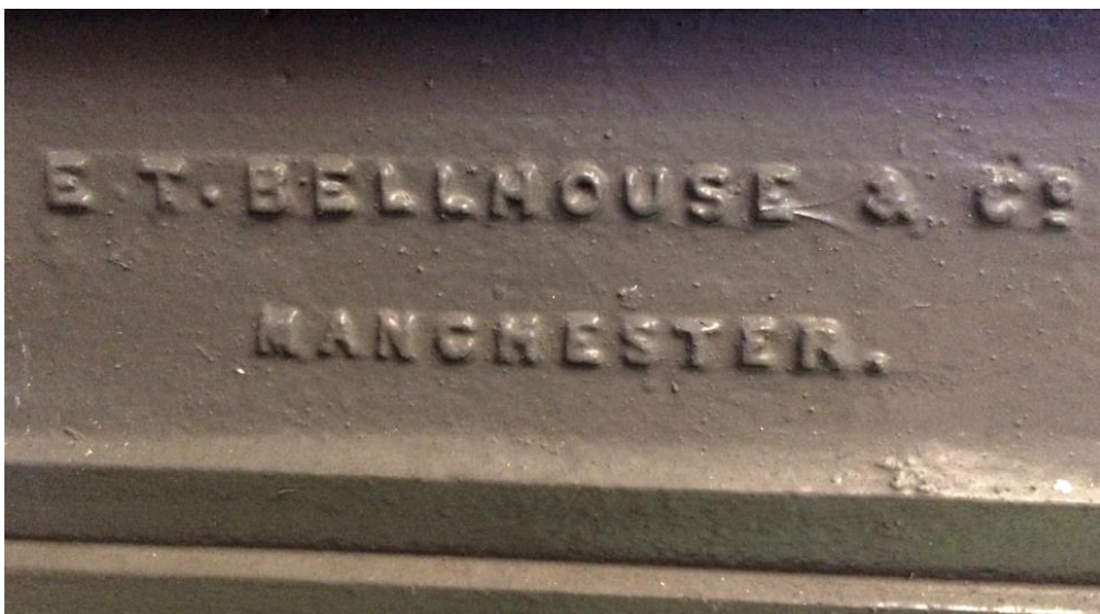
Figure 14: Original makers stamp on the bottom of a number of cast iron columns. (Source: SLHA January 2024)
