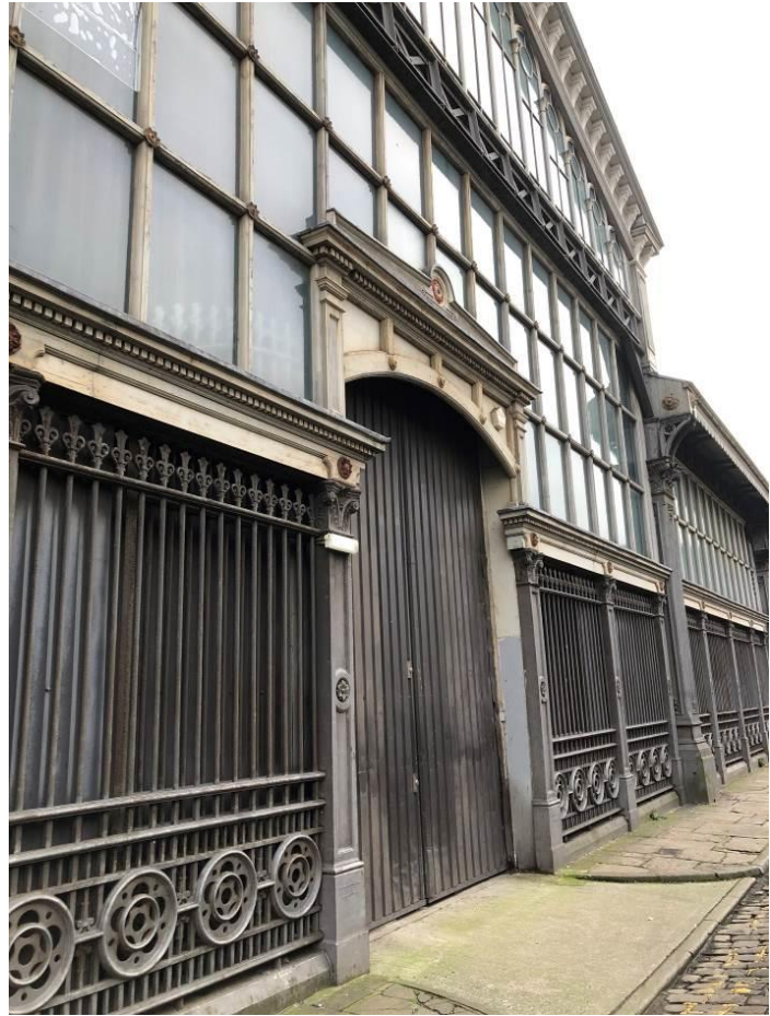
Figure 67: The central entrance to the west elevation on Barton Street, showing the only examples of surviving original cast iron railings to the bottom part (left and right). Although the central gates are modern, the original cast iron railed gates survive behind the corrugated metal within the side elevations.
