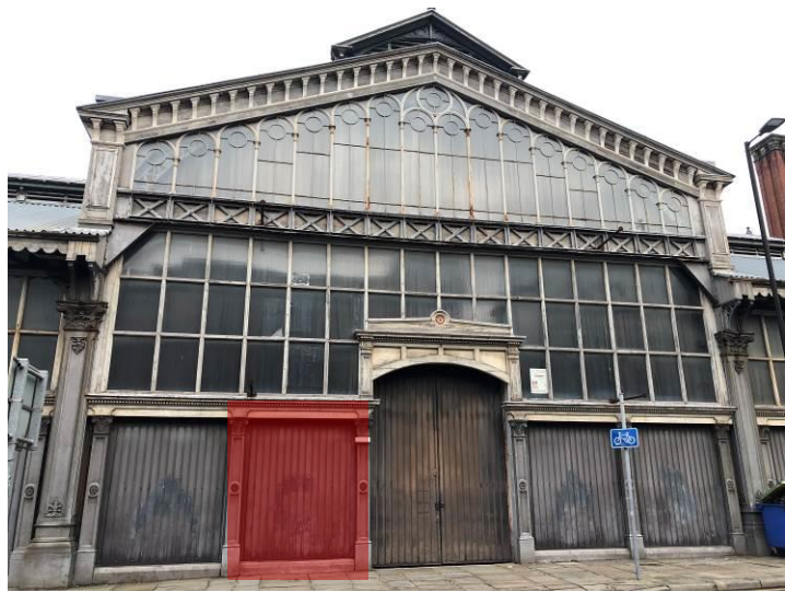
Figure 61: The central section of the south elevation, showing the original glazed framework with modern corrugated metal sheeting and gates. The shaded area denotes the location of the 1915 entrance cartway.
