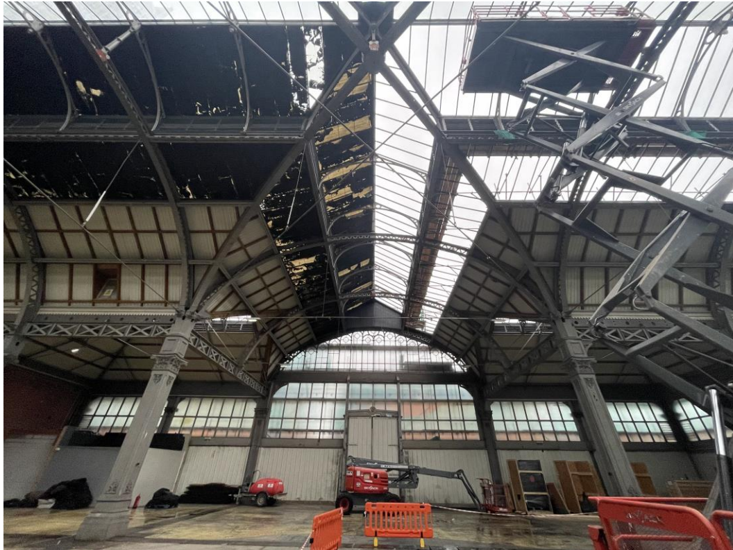
Figure 76: Looking south through the centre of the market towards the Liverpool Road elevation, showing the 1980s clear roof panels to the left compared by the current installation of new, clear glazing to the right.
