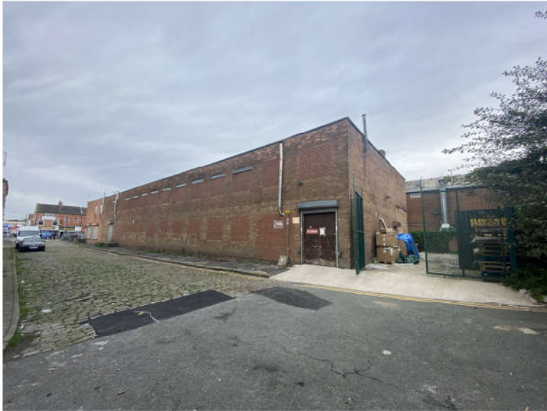
Looking West Towards Existing Building
