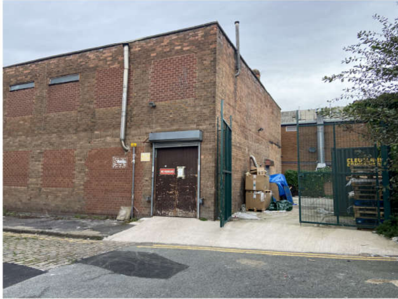
Looking Northwest Towards Site
