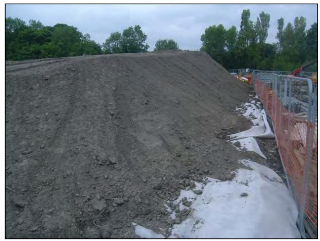
Photograph 6: Example of good stockpile management with soils placed on geotextile with fences to prevent accidental cross-mixing
