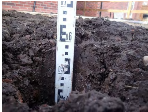
Photograph 4: Example validation photograph demonstrating depth of inert cover
