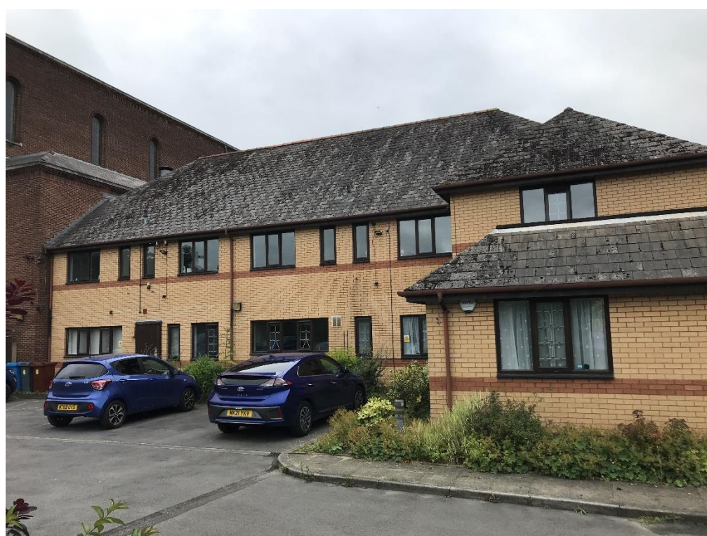
Photograph 2 – Left Hand Side Elevation
